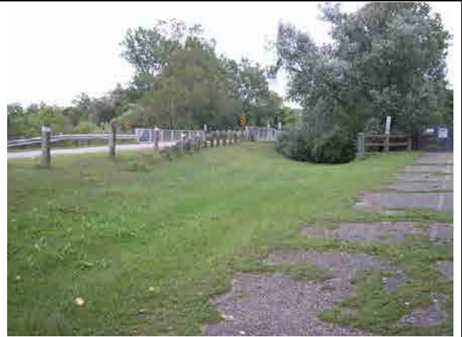
Photo #2 – Remnant of right upstream embankment (county roadway constructed after the dam is located immediately upstream).
