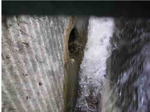
Photo #7 – Lehman Dam toe drain (inside the outlet structure) was observed to be functioning, draining left portion of the embankment.
