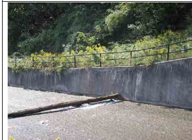
Photo #35 – Right downstream wingwall, middle portions. Note railing and brush vegetation at top of wingwall.
