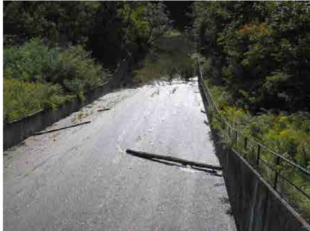
Photo #43 – Main spillway, looking downstream.
