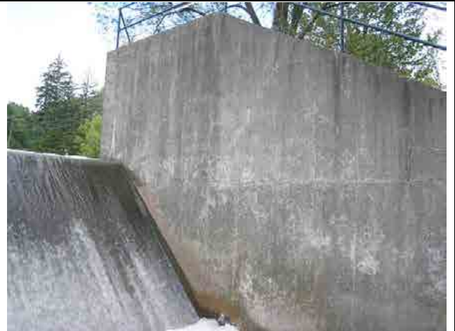
Photo #32 – Right downstream wingwall, in good condition.
