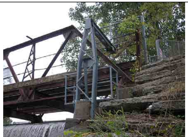
Photo #24 – Close up view of the upper portions of the left downstream wingwall, at the interface with the bridge deck.
