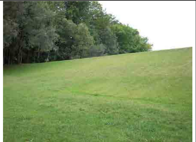
Photo #2 – Right downstream embankment, looking towards the right bank of the headpond.
