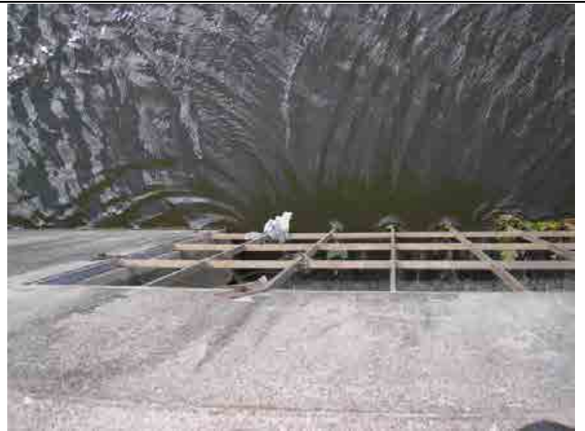
Photo #28 – Typical view at the intake grate. Small amount of trash observed adjacent to grate.
