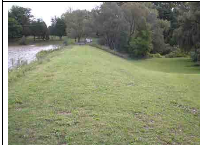
Photo #5 – Right embankment, looking towards the main structure. No evidence of cracking, seepage or loss of fill on the downstream side.
