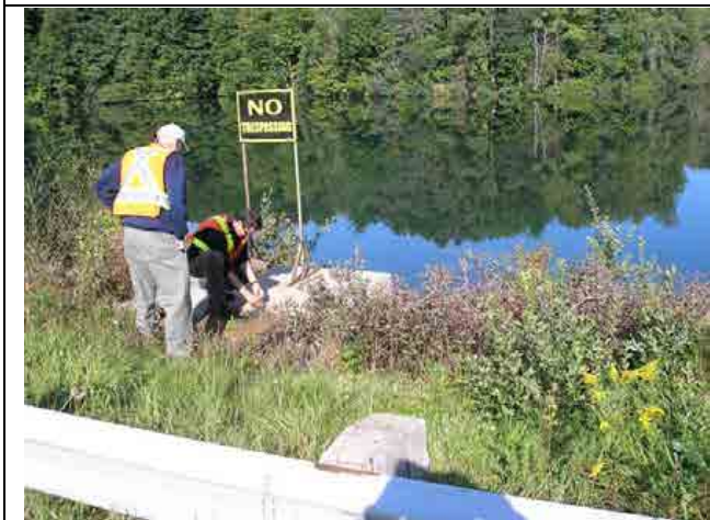
Photo #9 – Lift control chamber, located on top of left upstream embankment.
