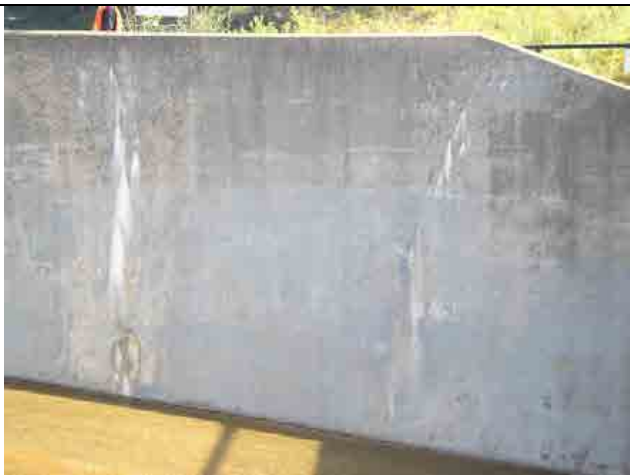
Photo #23 – Left upstream wingwall, closer to the roadway bridge.
