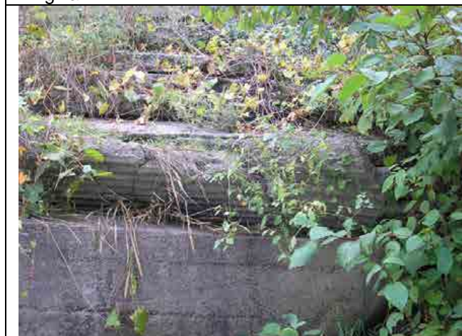
Photo #23 – Upper portions of the left downstream wingwall. Note the stacked blocks on top of the concrete wingwall.
