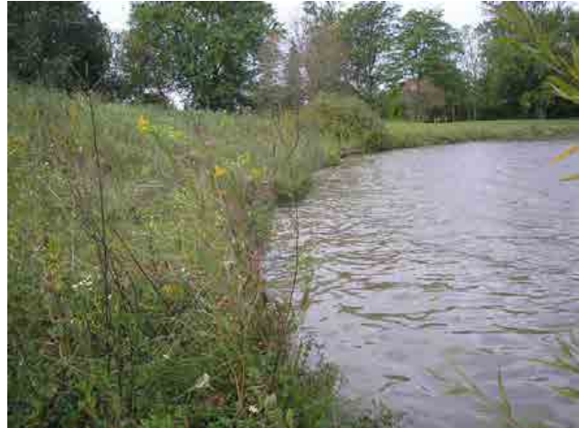
Photo #7 – Right upstream embankment, vegetated with tall grasses
