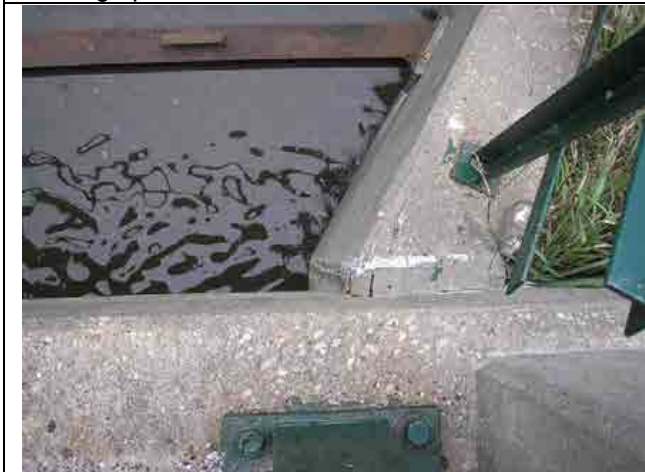
Photo #29 – Close up of the top view of the right downstream wingwall and bridge abutment.
