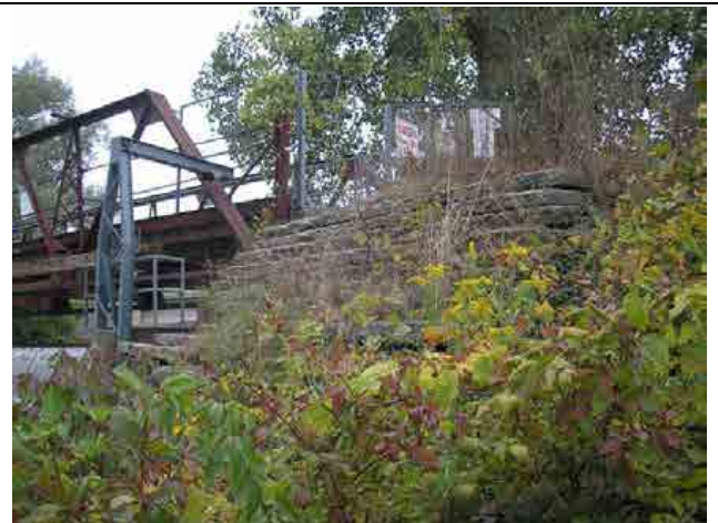
Photo #22 – Left downstream wingwall. Upper portions consist of stacked blocks, grouted together.
