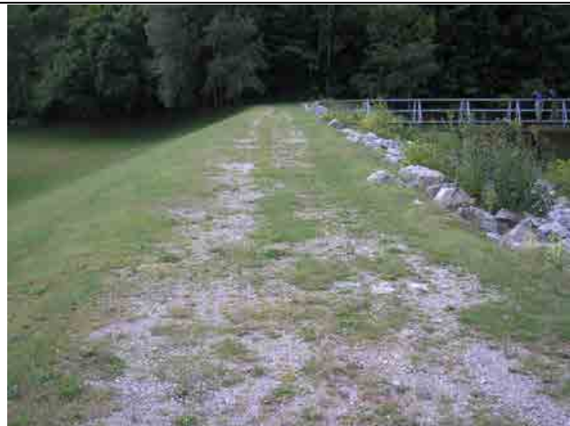
Photo #21 – Top of the embankment, standing near spillway and looking towards the right bank.
