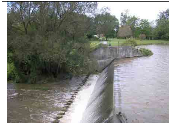
Photo #15 – Norwich Dam main spillway, looking towards the right wingwall. Note trees in close proximity to the right downstream wingwall.
