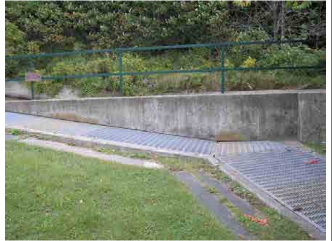
Photo #16 – Lower portion of the Lehman Dam fish ladder. The adjacent right downstream wingwall concrete is in good condition.
