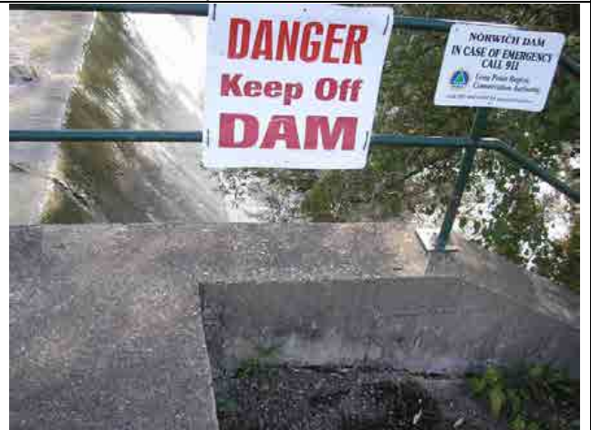
Photo #22 – Right downstream wingwall. Concrete appears in generally good condition. Some cracking noted at the wetwell-wingwall interface, on the downstream face.
