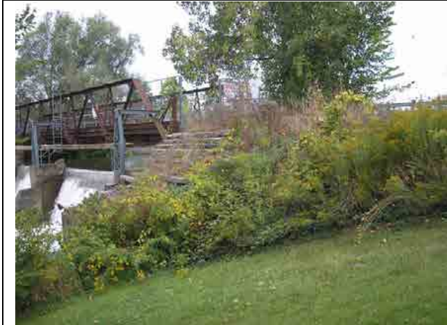
Photo #9 – Lower portions of the left downstream embankment. Parts of the embankment are covered with dense brush vegetation.
