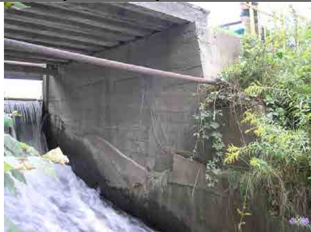
Photo #21 – Left downstream wingwall, underneath the bridge. Evidence of past concrete repairs is evident.
