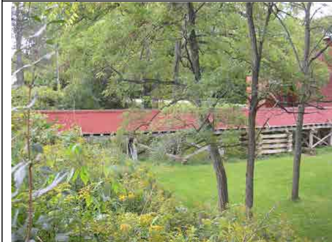
Photo #9 – Backus millrace is an elevated channel, supported by a timber pile bent structure.
