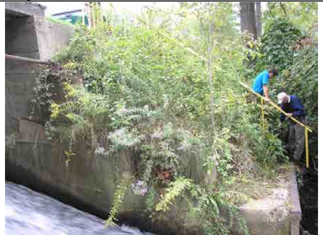
Photo #22 – Left downstream wingwall. Slope above consists of grouted concrete blocks, with brush vegetation growing between the blocks.
