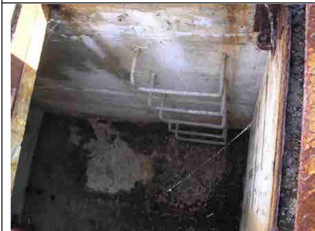
Photo #11 – Access to the lift chamber from above. Minor concrete deterioration at the top.
