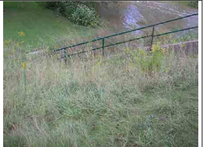
Photo #38 – Downstream slope of the left embankment, at the left downstream wingwall. Slope is vegetated with grass.
