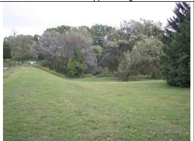
Photo #6 – Right downstream embankment. LPRCA staff notes that past dredge material was placed on top of embankment and adjacent downstream areas.
