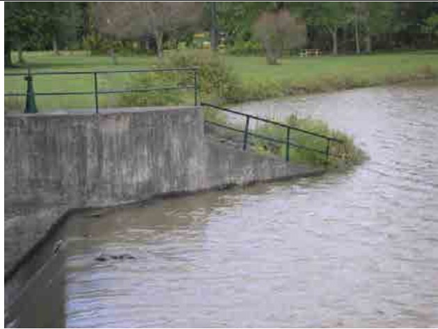
Photo #27 – Right upstream wingwall. Concrete appears in generally good condition.
