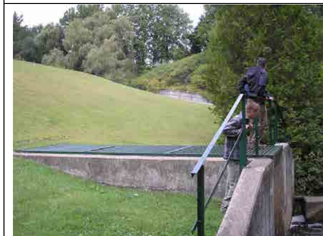
Photo #5 – Lehman Dam outlet structure, looking towards the spillway.
