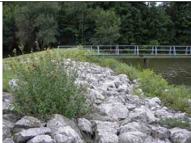
Photo #23 – Right upstream embankment, looking towards the right bank.
