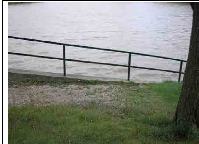
Photo #35 – Left upstream wingwall, looking towards the headpond.
