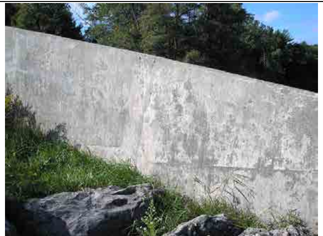
Photo #16 – Left upstream wingwall, along the upstream slope. Concrete is in generally good condition.
