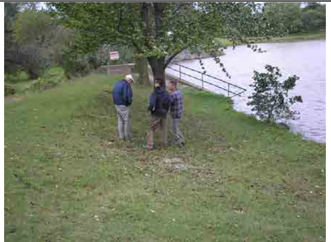
Photo #10 – A general view of the left embankment.
