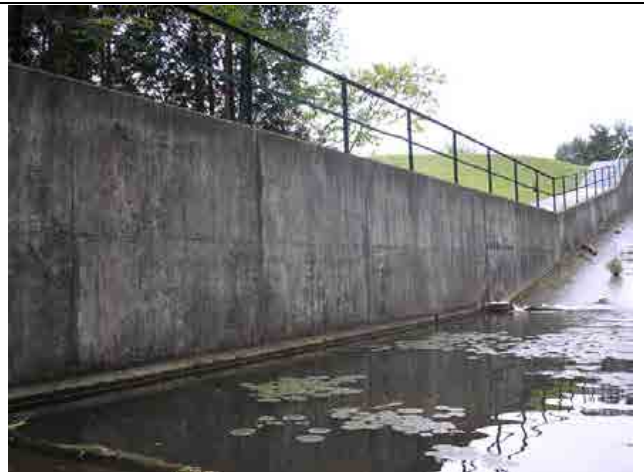
Photo #40 – Right downstream wingwall, as seen from the stilling basin. The wingwall also functions as the fish ladder channel.
