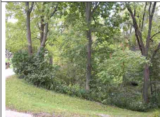
Photo #11 – Backus Mill Dam, right downstream embankment. Slope is approximately 1.5H:1V and is covered with heavy brush and mature trees. Seepage at toe of slope was not observed.
