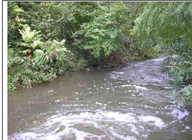
Photo #13 – Lehman Dam downstream channel. Banks heavily vegetated.
