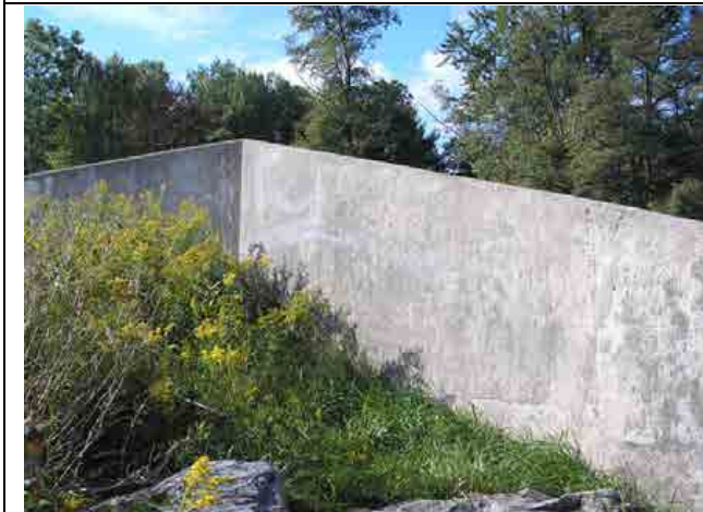
Photo #17 – Left upstream wingwall, at top of slope.
