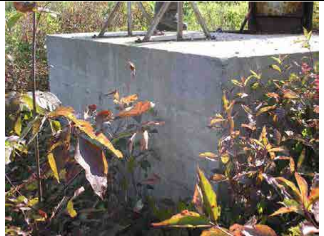
Photo #14 – Lift chamber, as seen from the left downstream slope.
