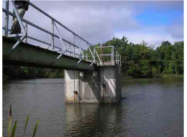
Photo #26 – Intake tower and access walkway, as seen from toe of embankment slope.
