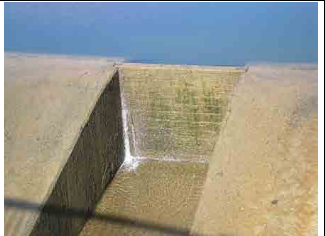
Photo #38 – Close up view of right stop logs.
