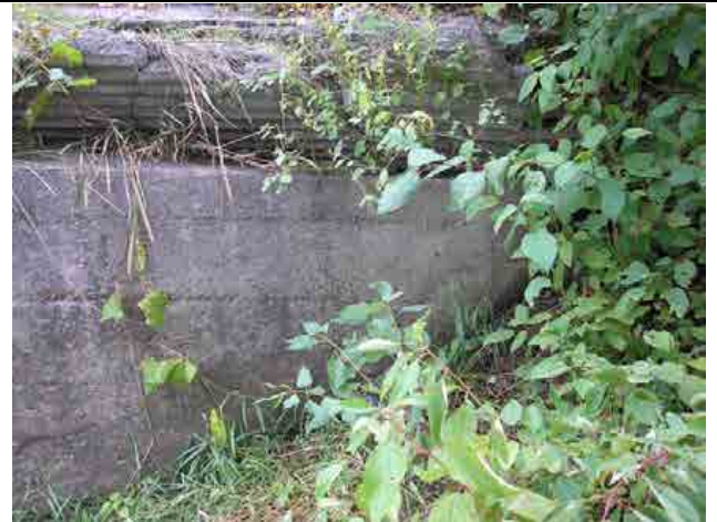
Photo #20 – Lower portion of the left downstream wingwall, at the interface at the bank.
