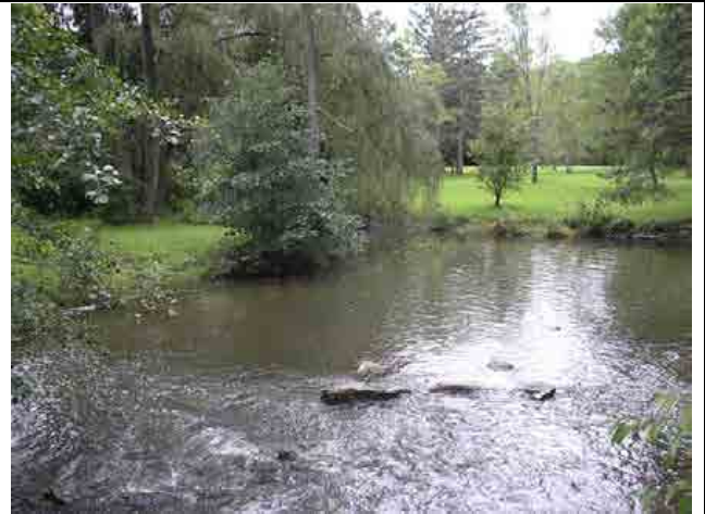
Photo #26 – Channel downstream of main spillway, some bank protection present.
