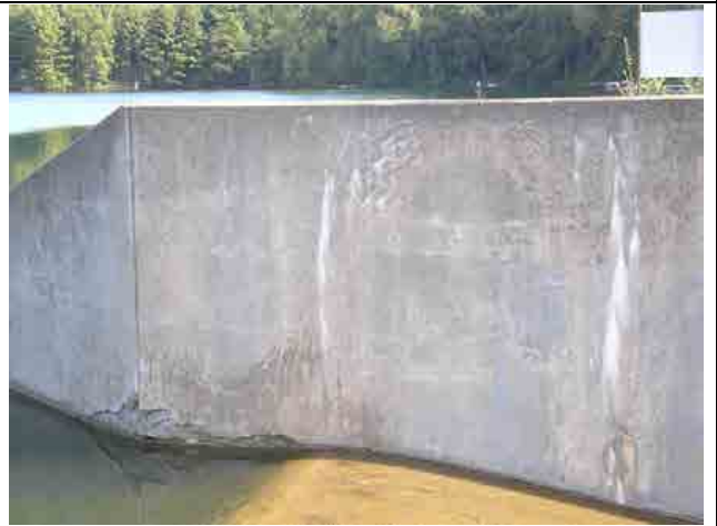
Photo #22 – Left upstream wingwall adjacent to the spillway.
