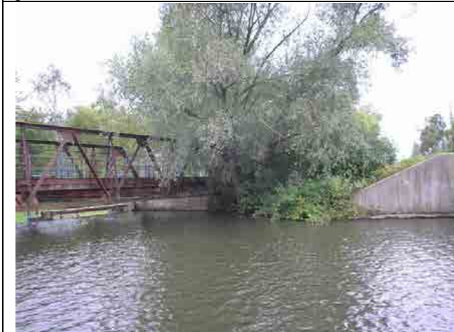
Photo #15 – Right upstream wingwall. Note tree growing adjacent to the wingwall.
