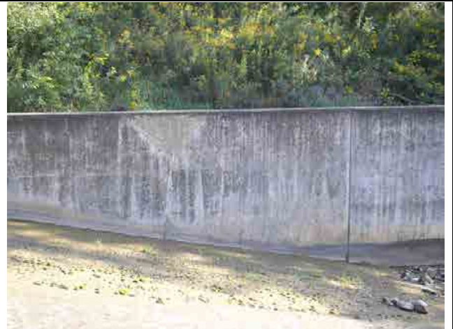
Photo #32 – Left downstream wingwall, panel 7.
