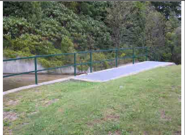
Photo #14 – Upper portion of the Lehman Dam fish ladder.
