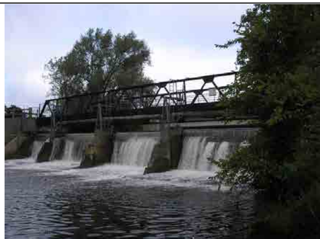
Photo #29 – Teeterville Dam as seen from the left downstream bank. The old roadway bridge is located on top of the dam, and carries maintenance traffic.
