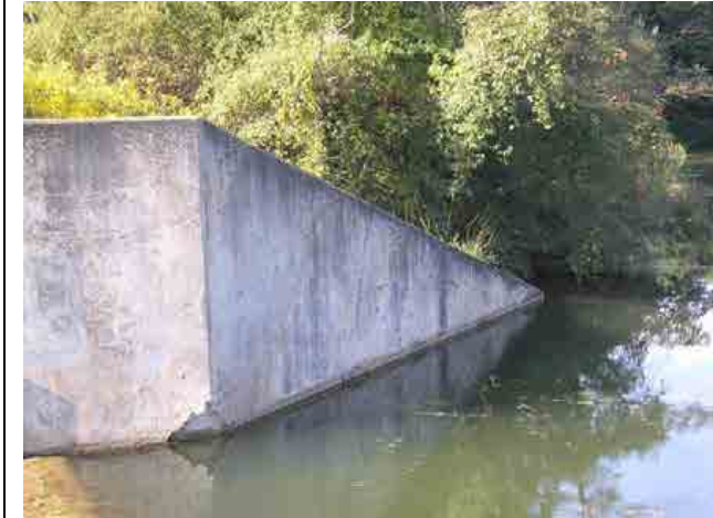
Photo #25 – Right upstream wingwall. Concrete is in generally good condition, although spalling is visible at waterline where wall changes alignment.
