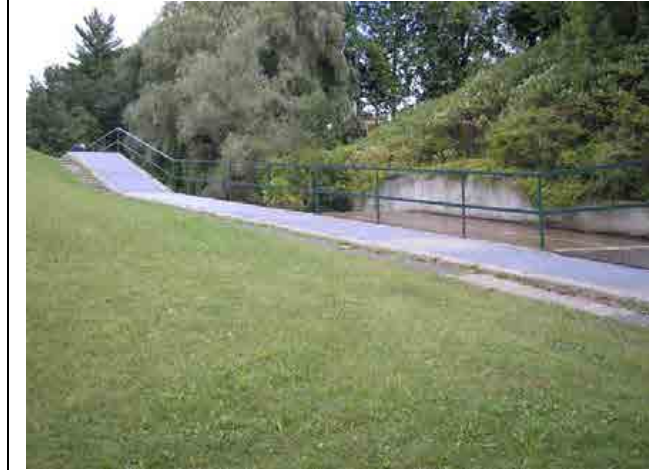
Photo #15 – Middle portions of the Lehman Dam fish ladder, as seen from the toe of slope.
