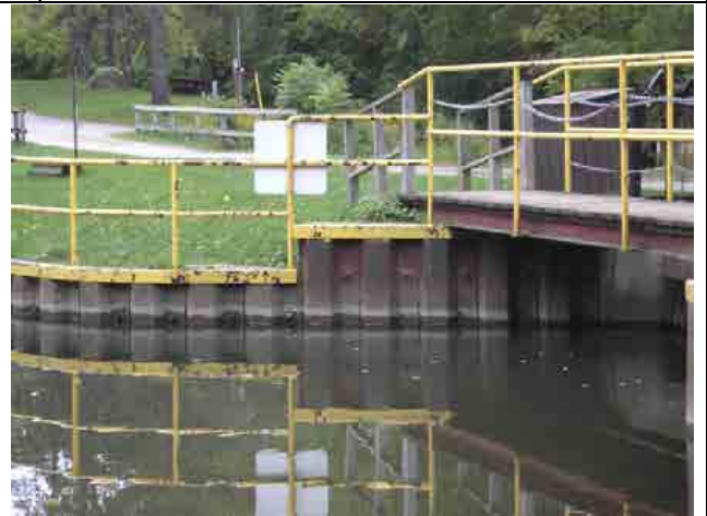
Photo #6 – Close up of the left upstream wingwall that consists of sheet piling. Piling is in good condition.
