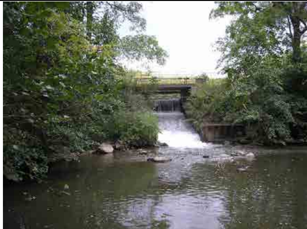
Photo #17 – Backus Mill Dam spillway, looking upstream.
