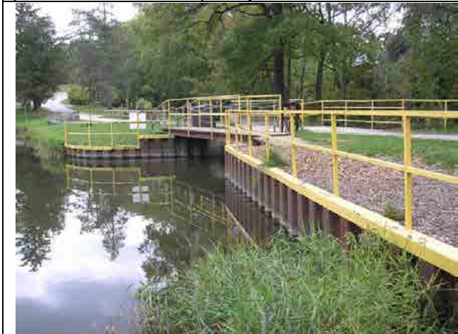
Photo #5 – Left and right upstream wingwalls at the main spillway structure.
