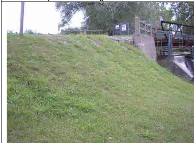
Photo #5 – Close up of the slope of the right downstream embankment.
