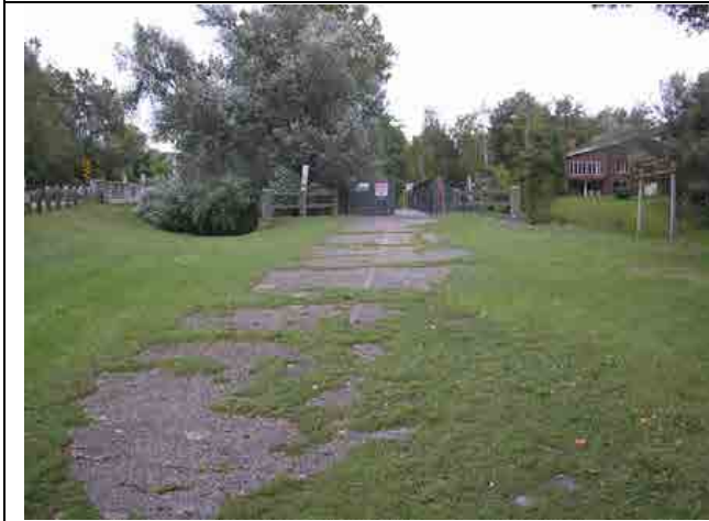
Photo #3 – Right embankment, looking towards the main structure. Surface of an abandoned road is visible on top of the existing embankment.
