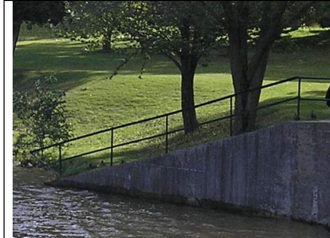
Photo #31 – Right upstream wingwall is in generally good condition.
