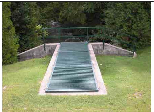
Photo #6 – Lehman Dam outlet structure, standing at toe of slope and looking downstream.
