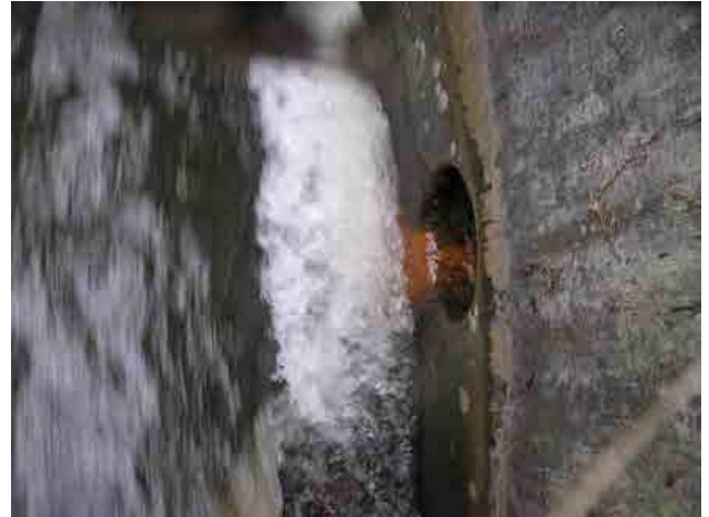
Photo #8 – Lehman Dam toe drain (inside the outlet structure) was observed to be functioning, draining right portion of the embankment.
