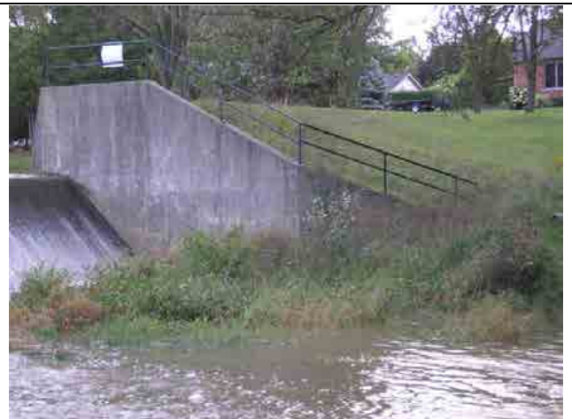
Photo #30 – General view of the right wingwall. Note the handrail and tall grass vegetation growing on the downstream site of stilling basin and wingwall.
