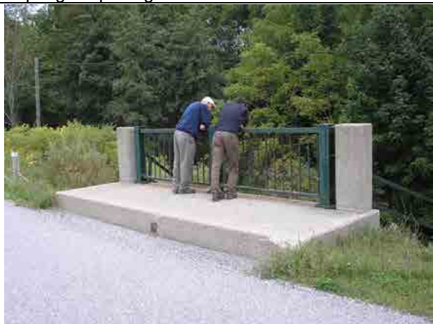
Photo #23 – Railing at the downstream side of the bridge.
