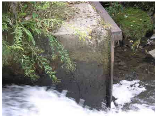
Photo #23 – Toe of left downstream wingwall consists of sheet piling, driven into creek bed. Downstream channel is covered with 100 mm riprap.
