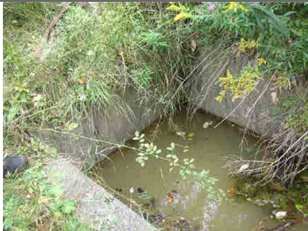
Photo #45 – Downstream low flow outlet structure. Area is generally vegetated with heavy brush.
