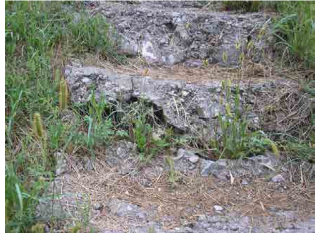
Photo #14 – Close up of the grouted portion of the right downstream slope, adjacent to the right wingwall.
