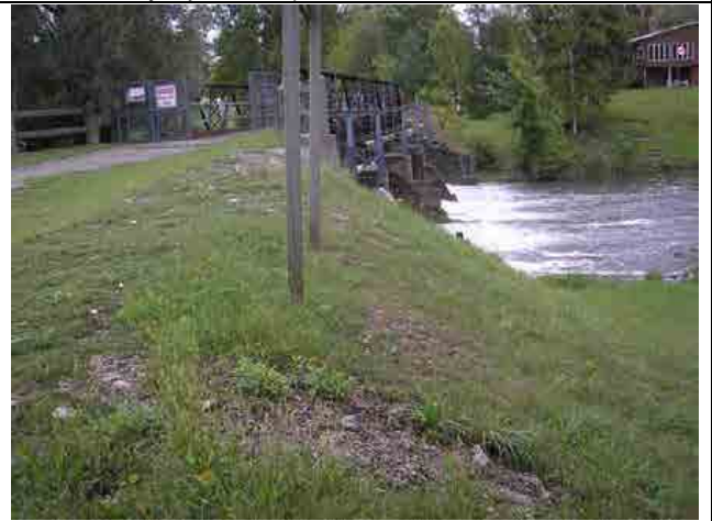
Photo #4 – Slope of the right downstream embankment appears in generally good condition, free of seepage.
