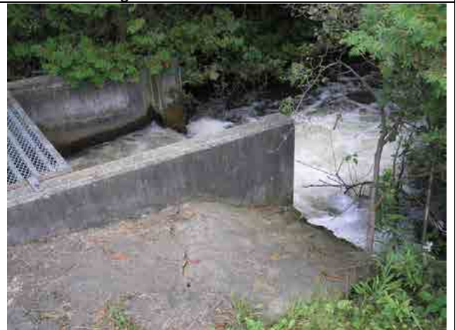
Photo #18 – Outlet of fish ladder, looking downstream. The channel immediately downstream of the outlet appears lower than bottom of outlet.
