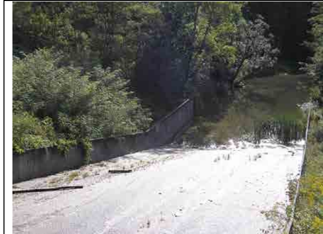
Photo #31 – Spillway and remaining left downstream wingwall panels.
