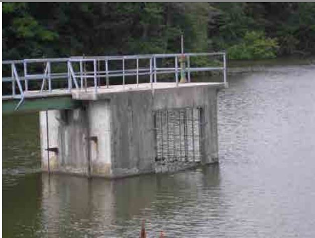
Photo #27 – Lehman Dam intake tower. Concrete is in generally good condition. Overflow gates are located on three sides of the structure.
