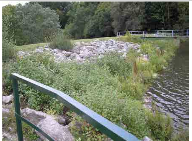
Photo #22 – Right upstream embankment. Some brush vegetation on upstream slope, which is lined with recently placed riprap above the waterline.
