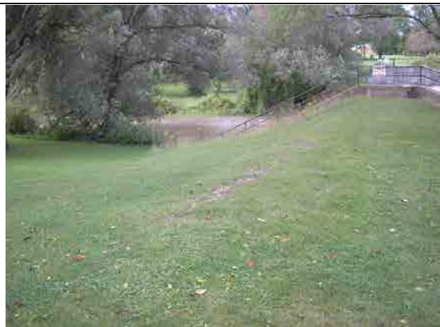
Photo #11 – Left downstream embankment, looking towards the main structure. Slope is grassed and free from evidence of seepage or erosion.
