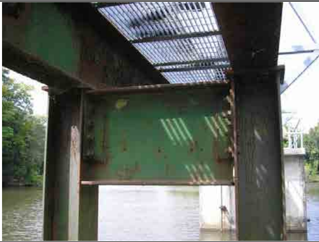
Photo #29 – Pile bent supporting the access walkway to the intake structure. Steel appears in good condition.
