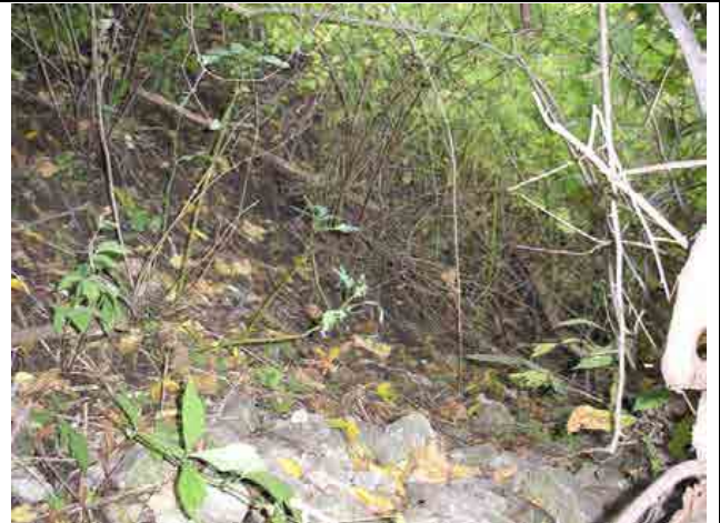
Photo #14 – Close up view of the left downstream embankment, showing riprap at toe of slope and brush vegetation.
