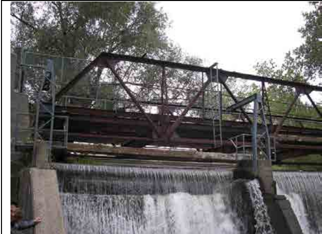
Photo #37 – Stop log lifting gantry cranes on the right most bay. Gantry cranes are anchored to the existing piers at each bay.
