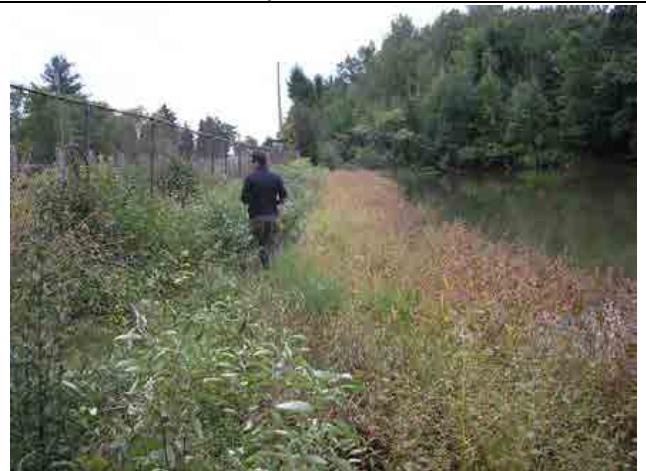
Photo #4 – Left upstream embankment. Upstream face lined with riprap, and overgrown with brush vegetation.
