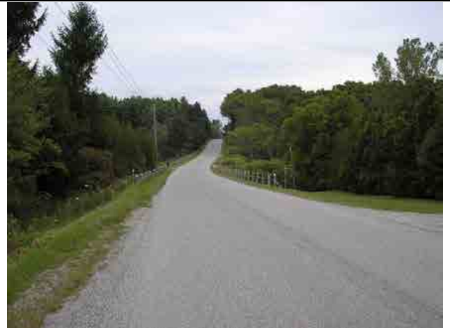
Photo #2 – Port Ryerse Road, looking from Woolley Road towards the Hay Creek Dam. Top of embankment is the asphalt road surface.
