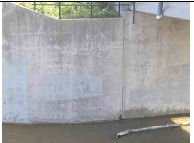
Photo #24 – Left upstream wingwall, at and underneath the roadway bridge. Concrete appears in good condition.
