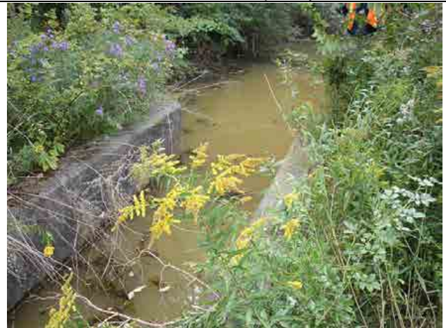
Photo #46 – Low flow outlet structure, looking downstream. Water depth measured as 1.5 m.
