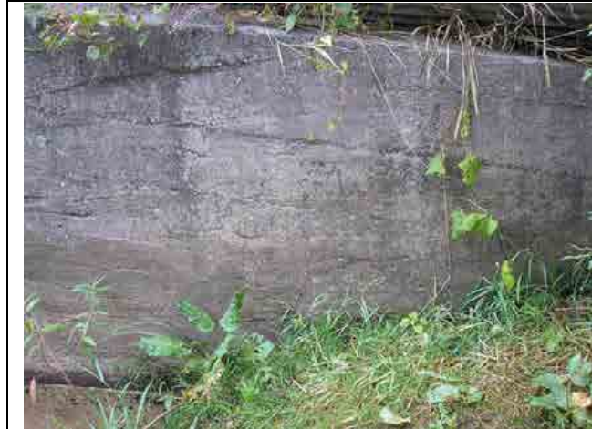
Photo #19 – Lower portion of the left downstream wingwall.
