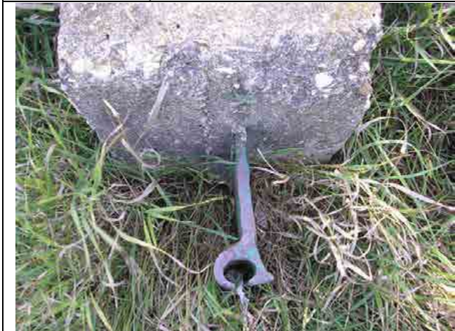
Photo #21 – Sheet pile embedded into concrete on the right wingwall.
