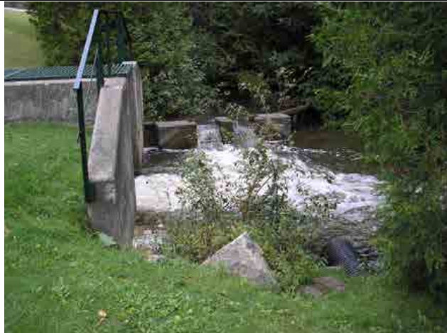
Photo #9 – Downstream outlet channel and fish ladder outlet. A perforated pipe observed for collecting upland storm water.
