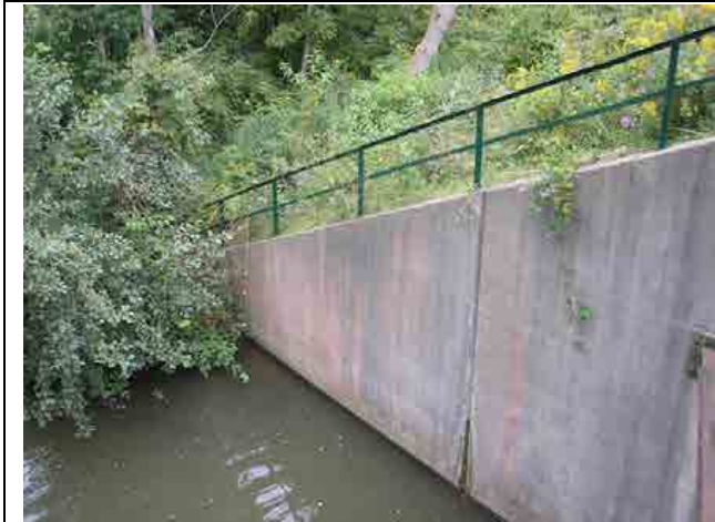
Photo #25 – Right upstream wingwall at Hay Creek Dam.
