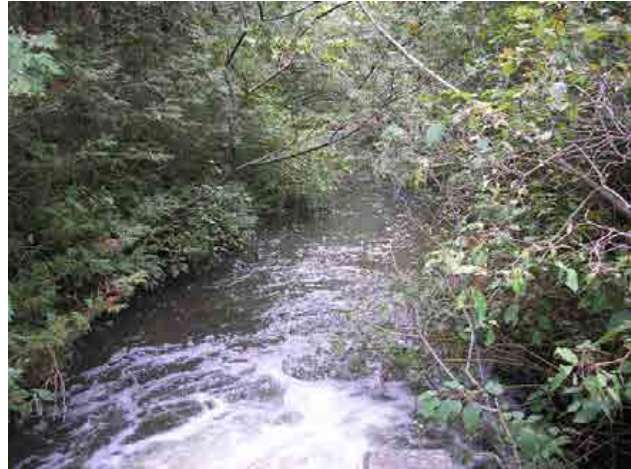
Photo #19 – Fish ladder outlet channel, looking downstream.
