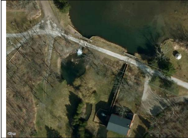
Photo #1 – Backus Mill Dam aerial photo 2006, downloaded from MNR Land Information Ontario database.
