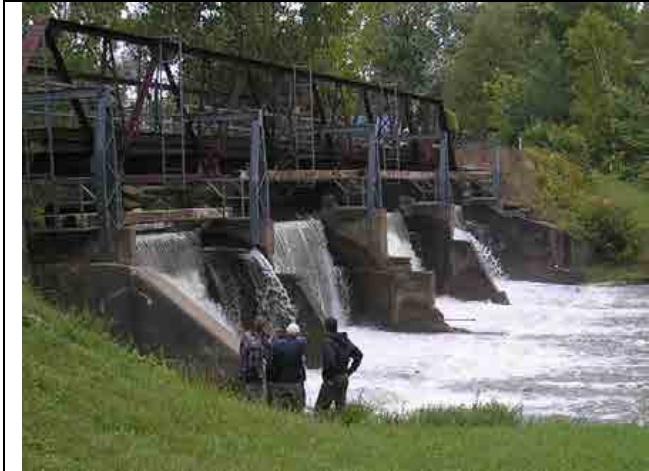
Photo #43 – Downstream channel, as seen from the right bank.
