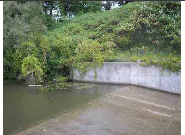
Photo #44 – Left upstream wingwall. Bank above wingwall covered with heavy brush vegetation.
