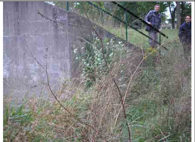
Photo #34 – Close up of right downstream wingwall, the downstream face.
