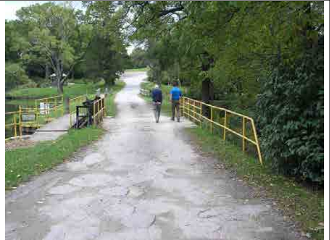
Photo #4 – Roadway crossing the dam, looking towards left bank. Existing roadway is surfaced with asphalt.
