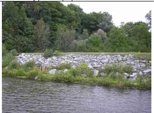
Photo #24 – Right upstream embankment, standing on intake structure and looking towards the left bank.
