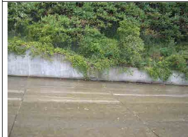
Photo #45 – Middle portion of the left downstream wingwall. Note vegetation above.
