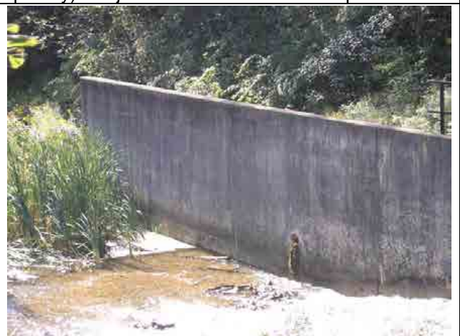
Photo #36 – Right downstream wingwall, panel 8. Corrugated steel toe drain is partially clogged, but still functional.
