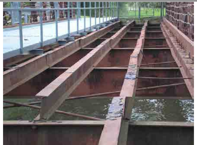
Photo #36 – General view of the stringers adjacent to the deck.
