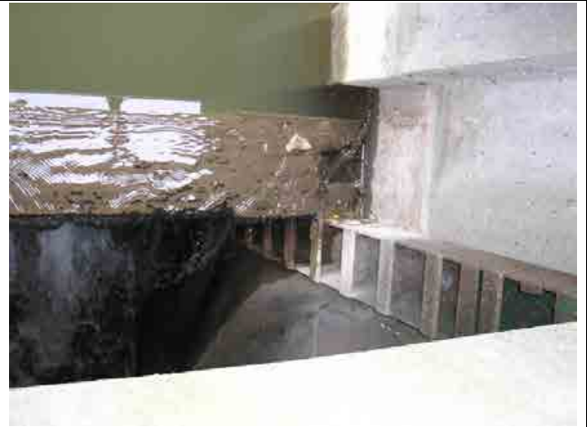
Photo #16 – Left gain, standing at top of control structure, looking down from the deck.
