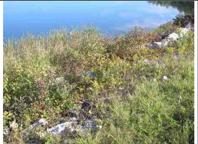
Photo #8 – Change in slope observed above the waterline approximately half way between the lift control chamber and the bridge.
