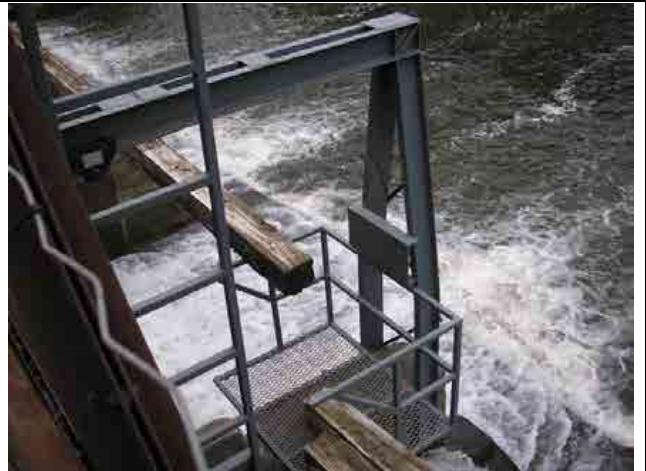
Photo #38 –Gantry crane as seen from the top of deck. Access to the gantry cranes is via ladder connected to the existing steel truss deck.
