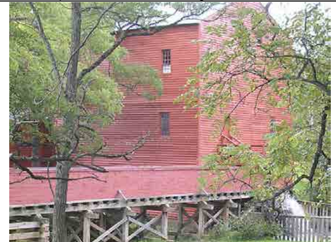
Photo #10 – Outlet of the millrace into the downstream channel.
