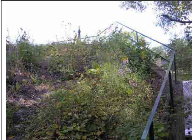
Photo #25 – Right downstream slope adjacent to right wingwall is vegetated with tall grasses. Note the handrail on top of wingwall.
