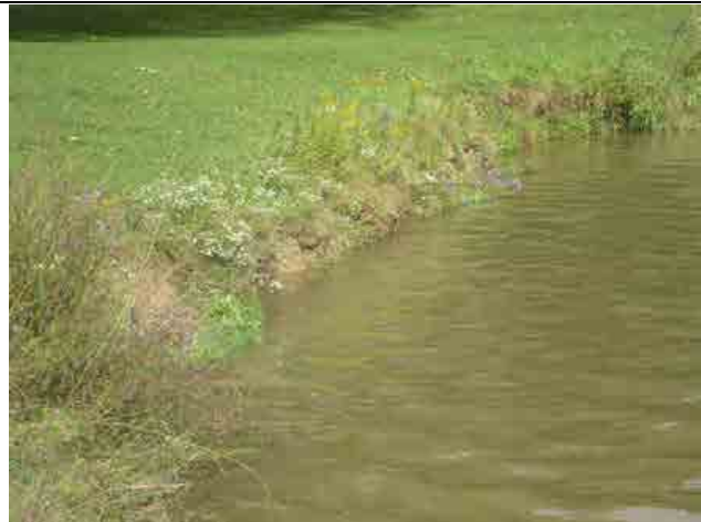
Photo #9 – Close up of the right slope on the right upstream embankment near the waterline.
