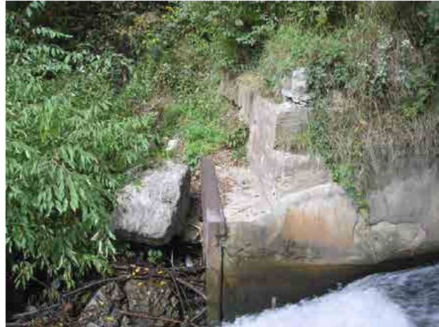
Photo #19 – Toe of the right downstream wingwall consists of sheet piling. Upper portions of the slope above wingwall consist of grouted concrete blocks.
