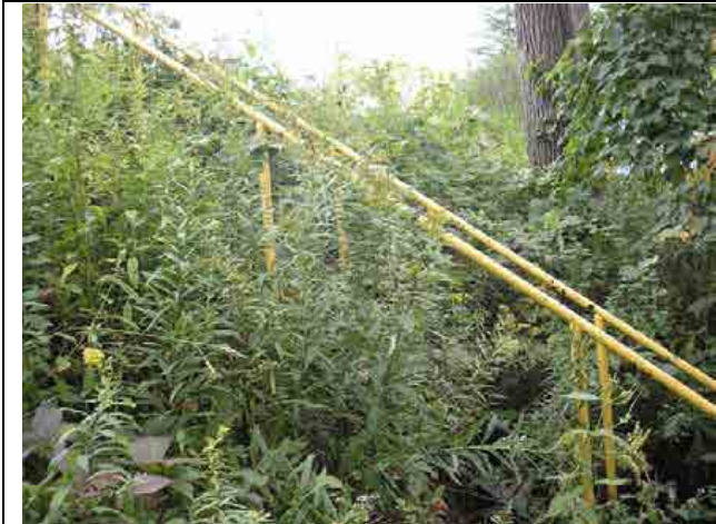
Photo #13 – Left downstream embankment, standing at spillway structure and looking towards the millrace. Slope is steep and covered with brush and mature trees.
