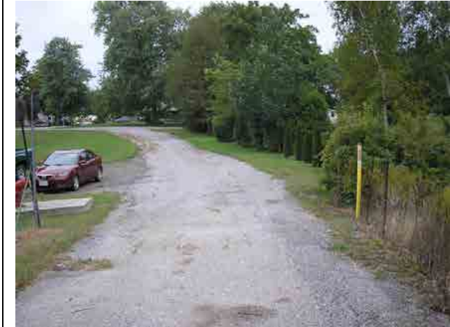
Photo #7 – Left embankment, standing at the dam looking eastward.
