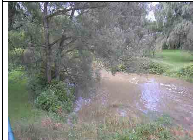
Photo #39 – Downstream channel, standing on left wingwall and looking downstream.
