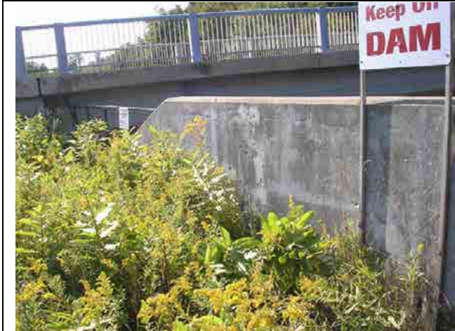
Photo #19 – Upper portions of the left upstream wingwall, just downstream of the Road 45 bridge.
