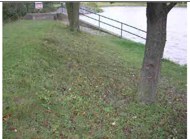
Photo #12 – A close up view of the left upstream embankment, noting the mature trees on the upstream slope.
