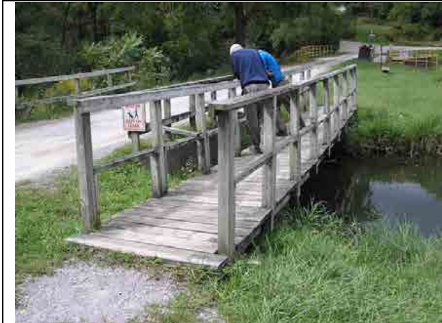
Photo #7 – Upstream embankment and millrace intake. Slopes of upstream embankment are fairly mild. Note pedestrian access over millrace intake.
