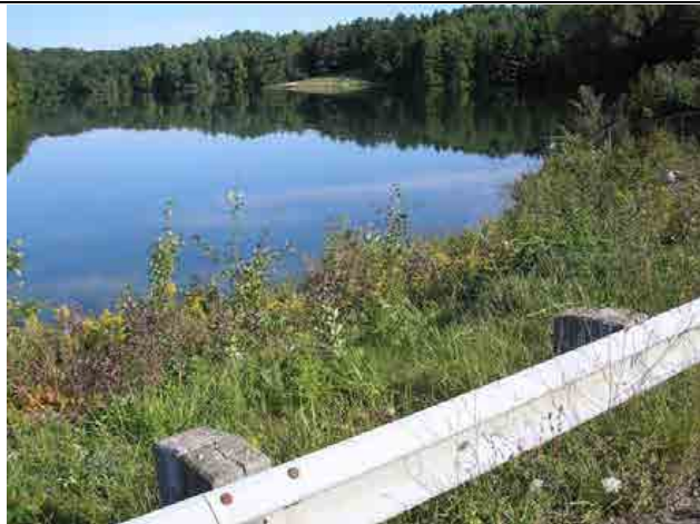
Photo #3 – Deer Creek headpond, standing on the left downstream embankment, looking towards the park area on the left bank.
