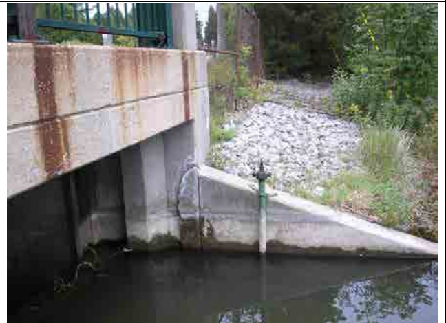
Photo #18 – Right upstream wingwall. Note the low flow gate opening mechanism. LPRCA staff confirms mechanism is operational.
