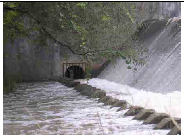
Photo #16 – Norwich Dam stilling basin. Note the outlet pipe located on the bottom of the right downstream wingwall.
