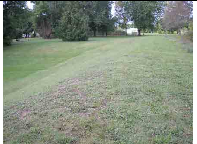
Photo #4 – Right downstream embankment, standing on right upstream wingwall, looking westward. Embankment appears in good condition.
