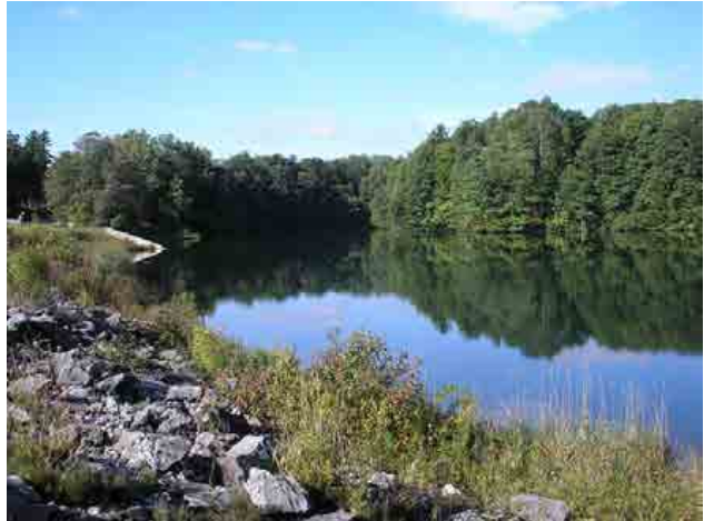
Photo #2 – Deer Creek headpond, standing on the left downstream embankment, looking towards the main structure.
