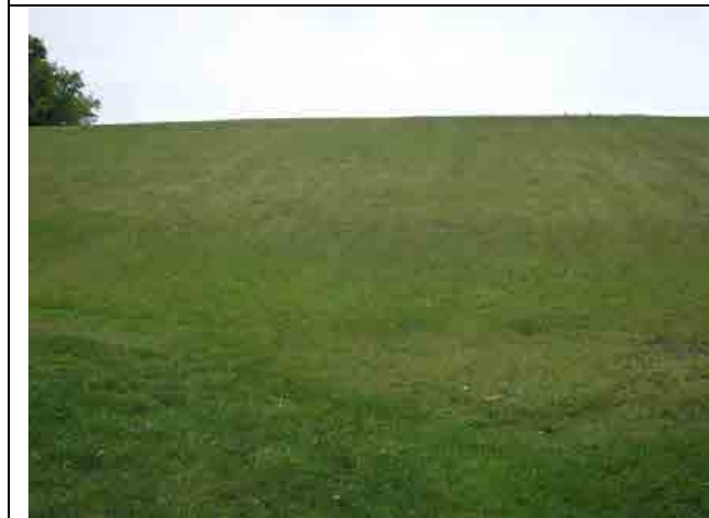
Photo #3 – Middle portion of the right downstream embankment.
