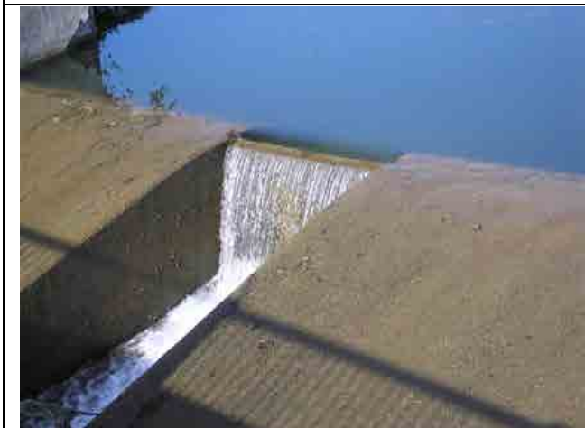
Photo #39 – Close up view of left stop logs.
