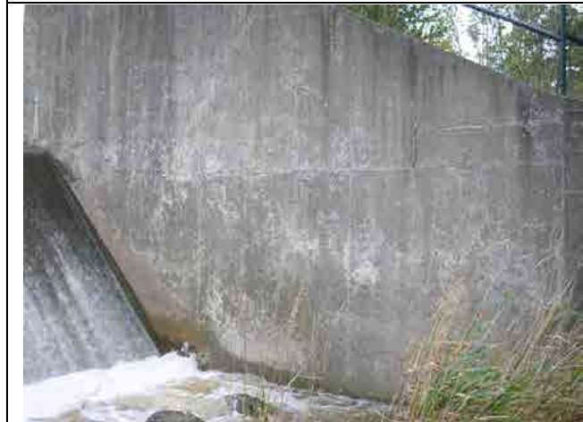
Photo #33 – Close up view of the right downstream wingwall.
