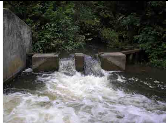
Photo #12 – Outlet of the fish ladder channel, Concrete blocks and sheet pile wall in good condition.
