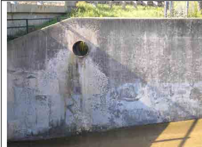
Photo #27 – Right upstream wingwall. Note the drain pipe that is the outlet of the ditch running parallel to the road.
