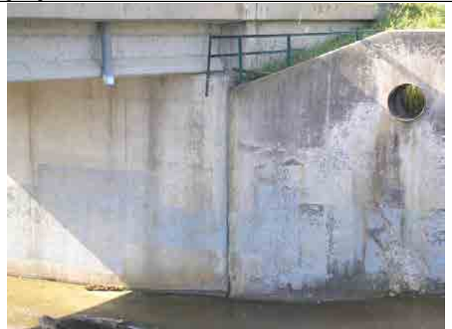
Photo #28 – Right upstream wingwall, underneath the existing bridge.
