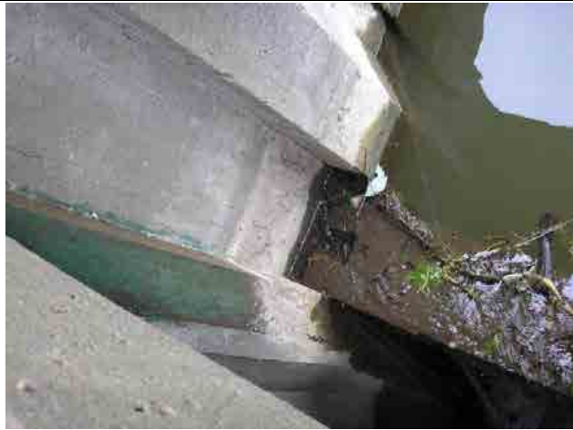
Photo #15 – Right gain, standing at top of control structure, looking down from the deck.
