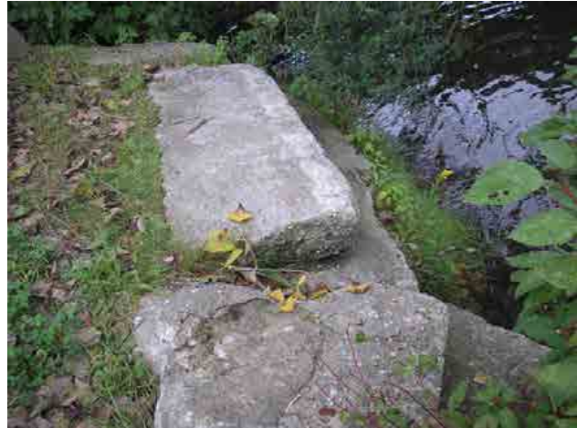
Photo #25 – Left upstream wingwall consists of stacked blocks, likely on top of poured concrete wingwall underneath.
