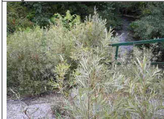
Photo #11 – Left downstream embankment, looking towards toe of slope. Portion of the embankment adjacent to left downstream wingwall is surfaced with asphalt.
