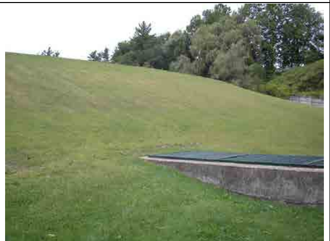
Photo #4 – Right downstream embankment, looking towards the spillway.
