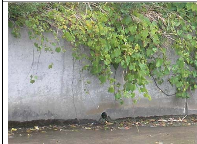
Photo #47 – Drain holes at the left downstream wingwall observed as functioning.
