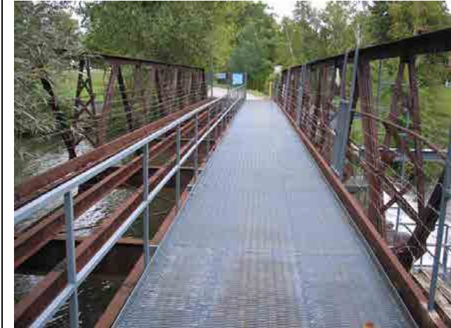
Photo #31 – Deck of the existing steel truss bridge. Decking is fairly new, and is supported by original steel stringers, girders, and trusses.
