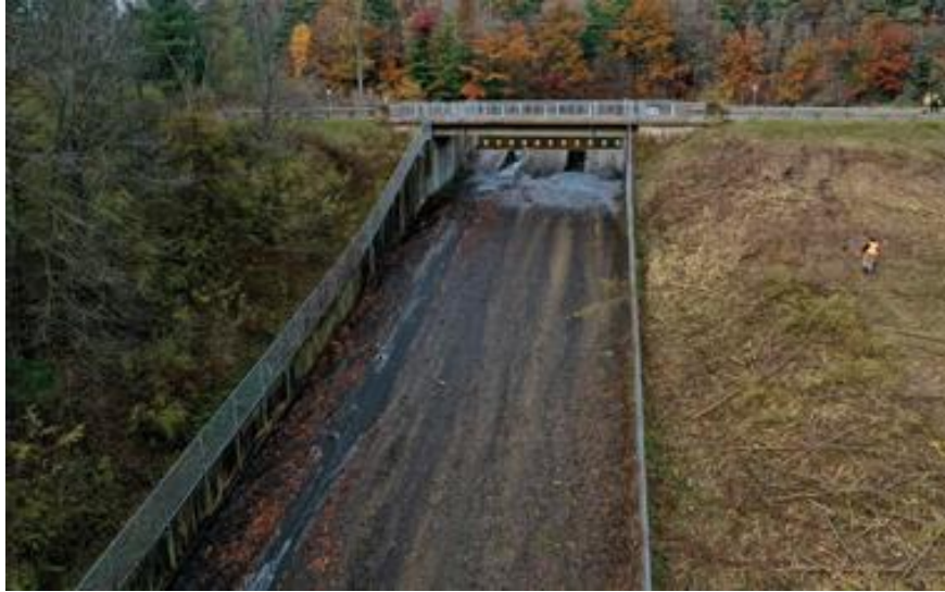
Figure 5: The upper portion of the dam's spillway
