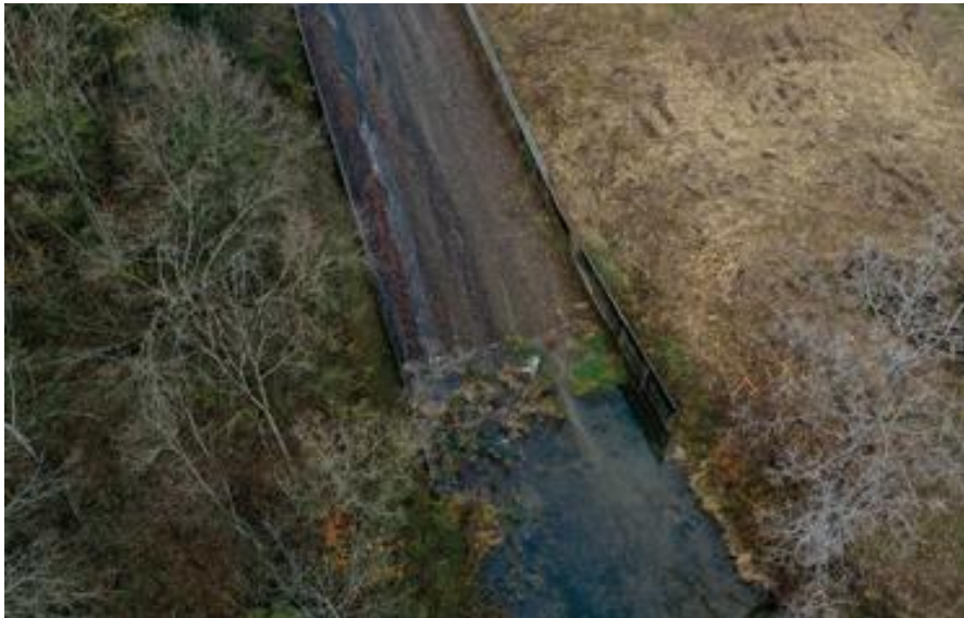
Figure 6: The lower portion of the dam's spillway
