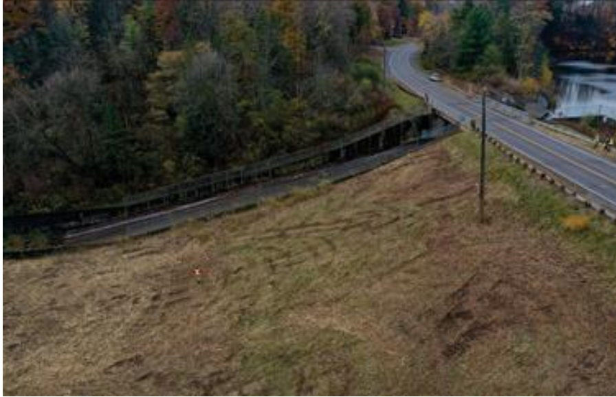
Figure 7: The downstream embankment of the dam
