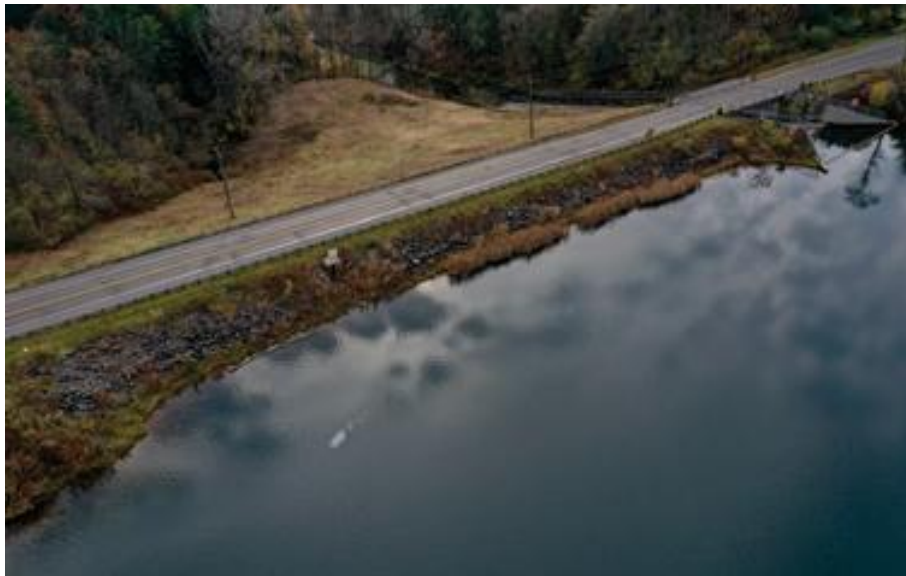
Figure 4: The upstream embankment of the dam
