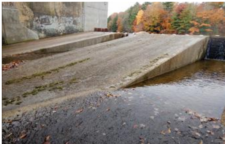
Figure 2: The dam's inlet looking upstream
