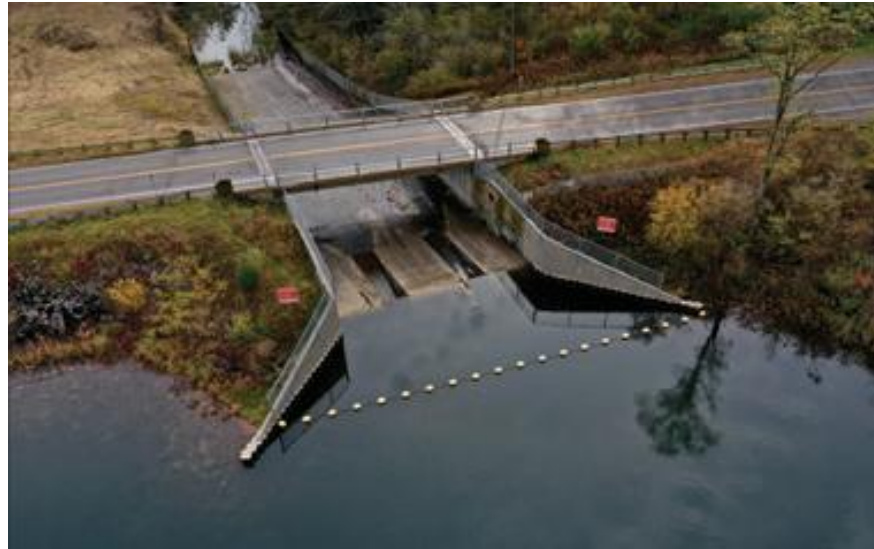
Figure 1: Upstream of the dam
