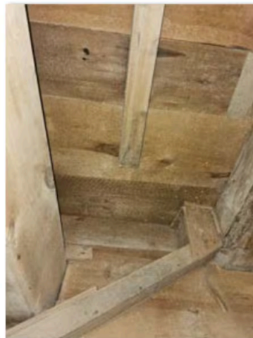
Image 14: Bending floor boards below equipment
