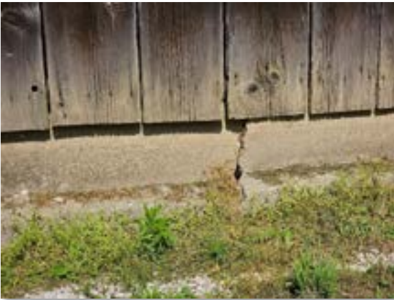
Image 21: Cracked foundation
