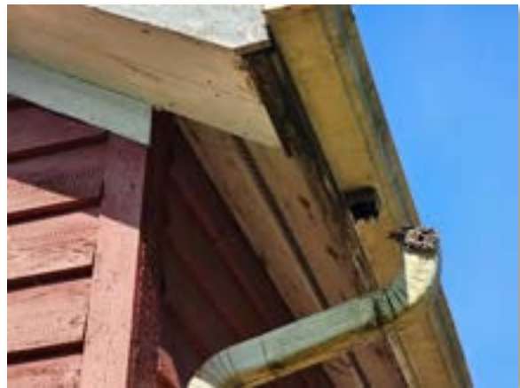
Image 50: Damaged downspout
