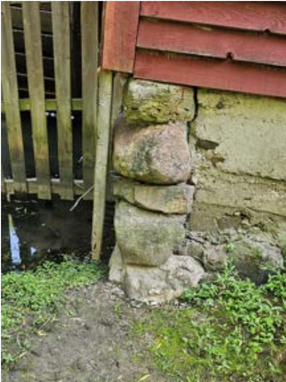
Image 9: Cracked foundation, South West Corner
