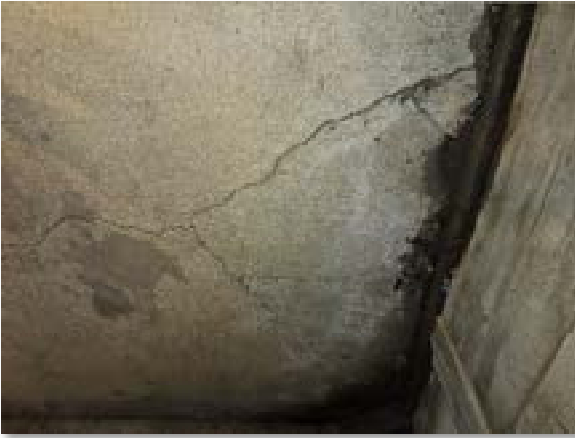
Image 27: Cracked foundation - Basement
