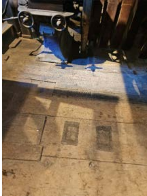
Image 18: Deflecting main floor framing Main floor level near equipment
