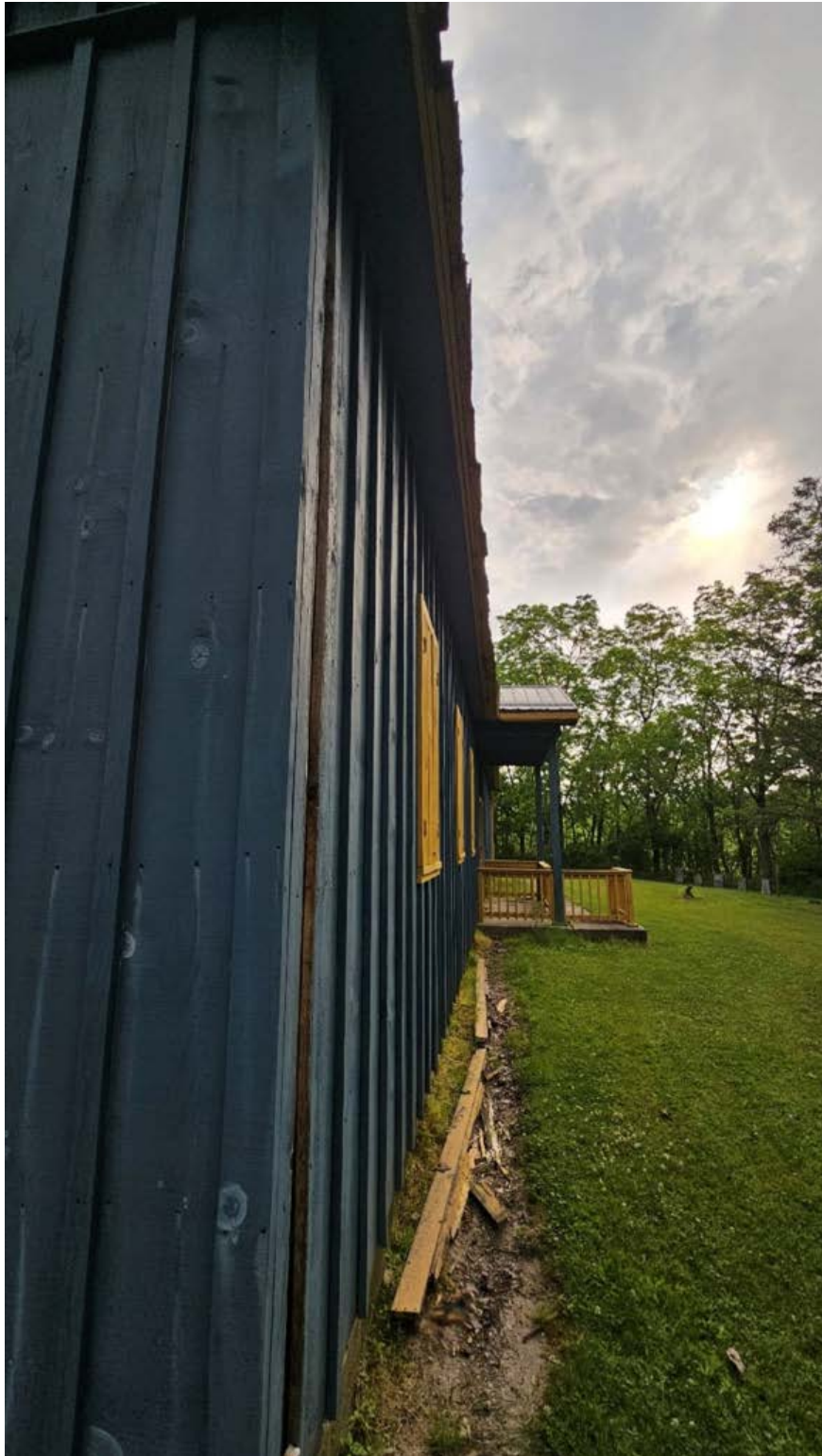
BUILDING 8 – MUSEUM – FAILED/ROTTED EAVESTROUGH AND EROSION
