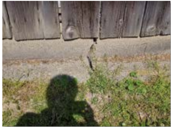
Image 22: Cracked foundation
