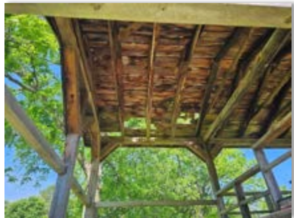
Image 39: Damaged Roof and Framing
