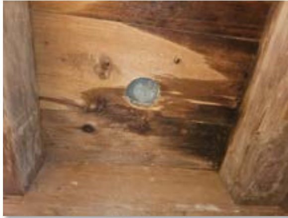
Image 28: Moisture at main floor framing, North Wall
