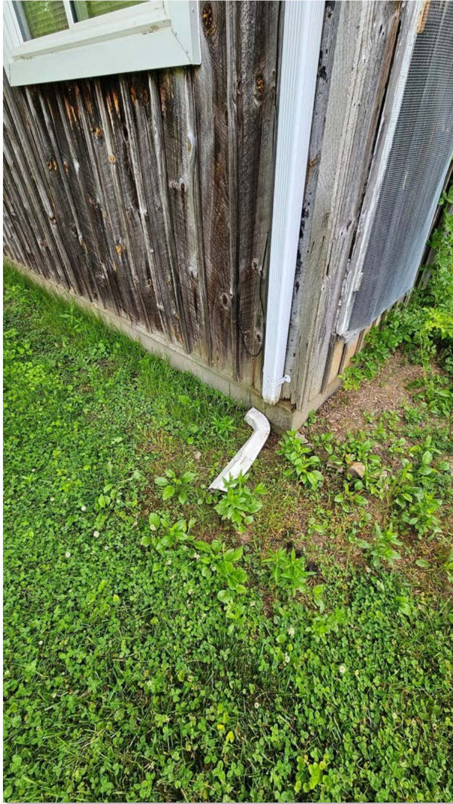
BUILDING 4 – HOMESTEAD – DISCONNECTED DOWNSPOUTS
