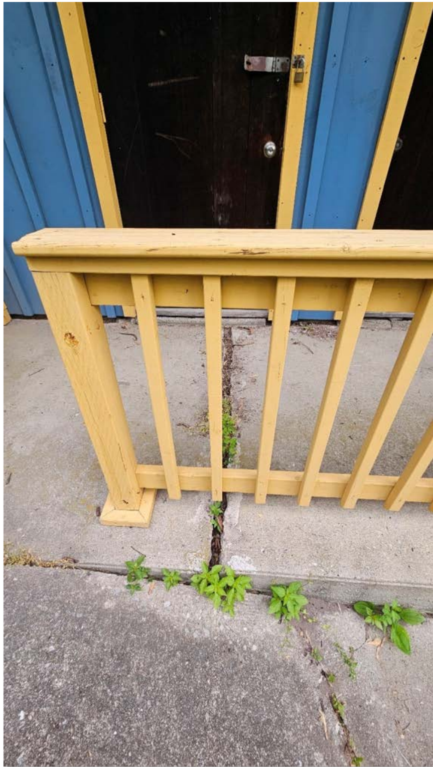
BUILDING 8 – MUSEUM – CRACKED CONCRETE
