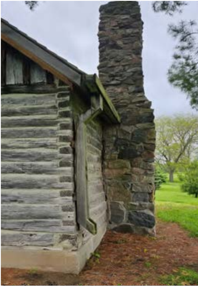
Image 63: Cracked fireplace chimney and eave trough drainage.
