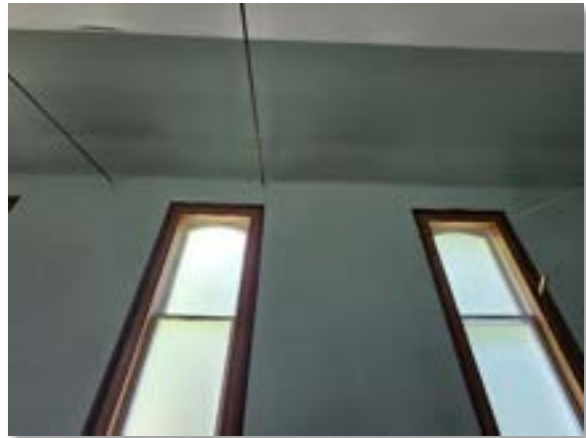
Image 75: Plaster Cracking at tie rod locations
