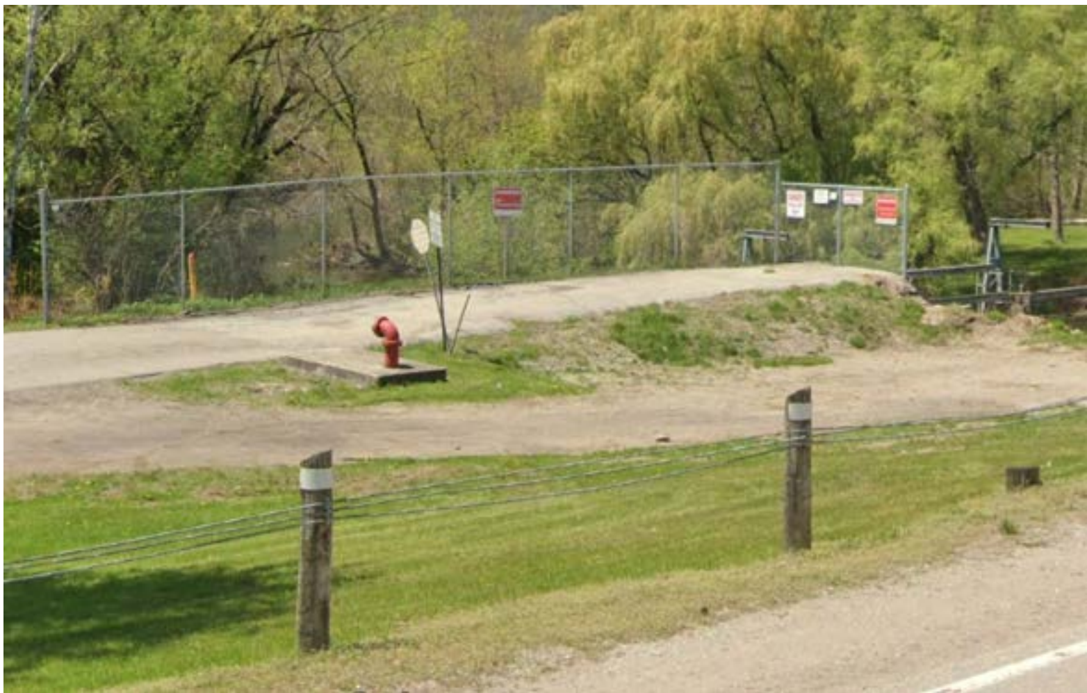
Dry Hydrant Adjacent Dam, Source: Montrose Environmental
