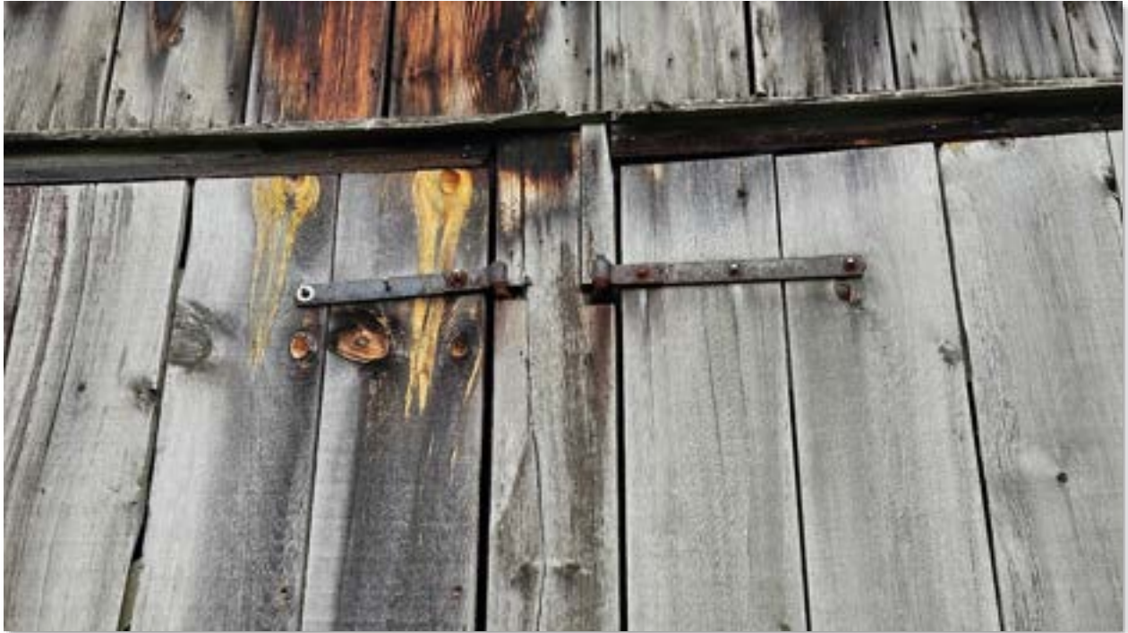
BUILDING 6 - FORBES BARN – FAILING HARDWARE
