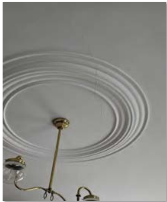
Image 14: Cracking in ceiling plaster on main floor.
