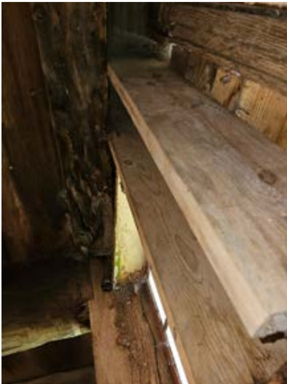
Image 29: Moisture along North Wall
