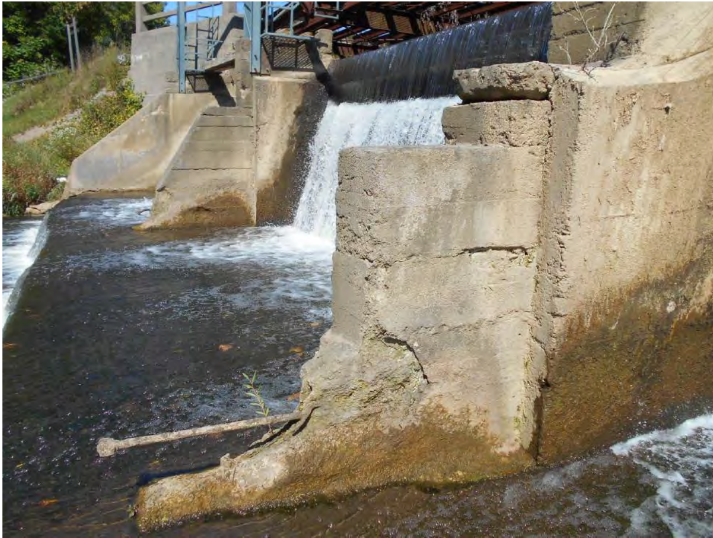
Concrete Deterioration @ Pier - Source: AECOM, 2015
