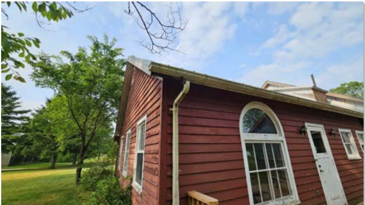
BUILDING 14 – STOREFRONTS – DISCONNECTED DOWNSPOUTS
