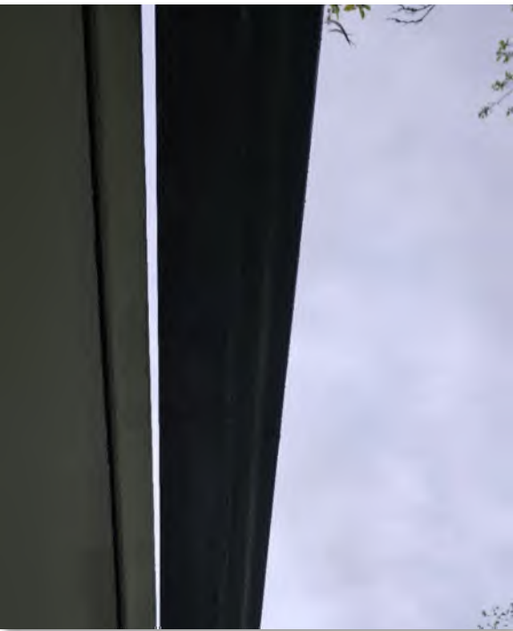
Image 13: Gutter gaps to fascia.
