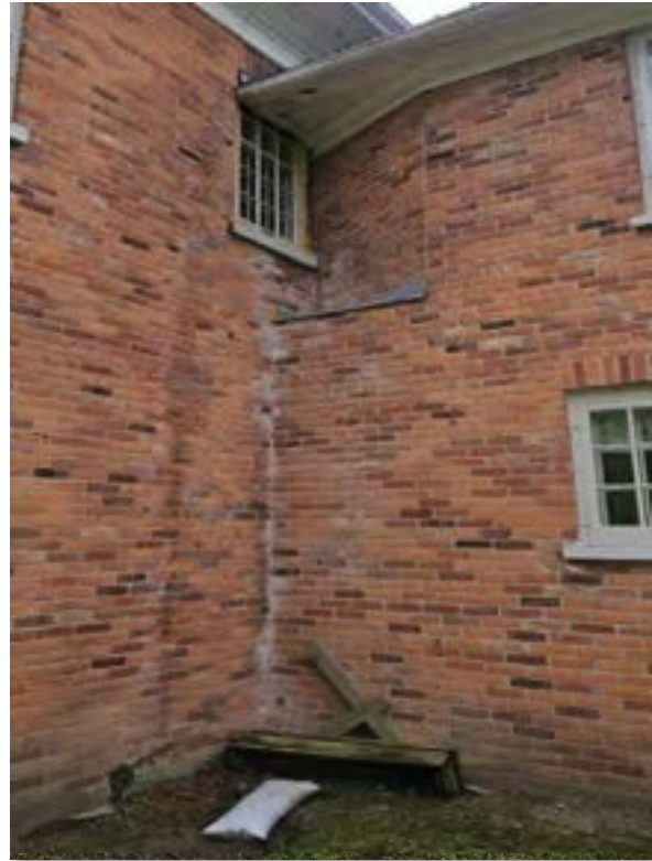
Image 7: Damaged Brick, Soffit and poor drainage at North side of building.
