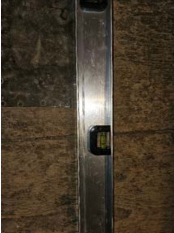
Image 17: Deflecting main floor framing Main floor level near equipment
