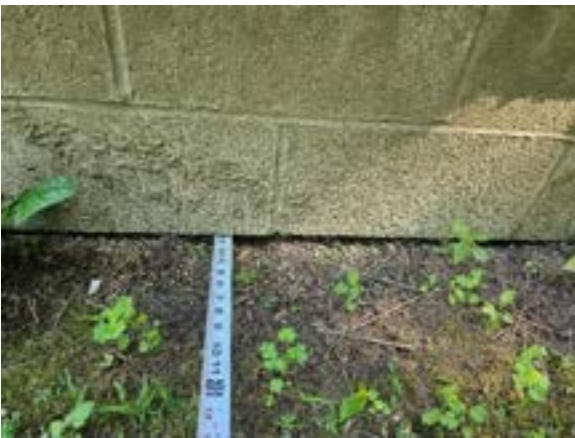
Image 72: Foundation wall offset and cracked
