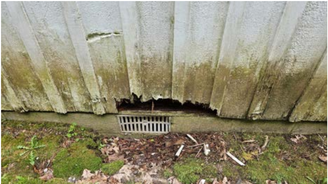
BUILDING 24 - TEETERVILLE CHURCH - ROTTED SIDING
