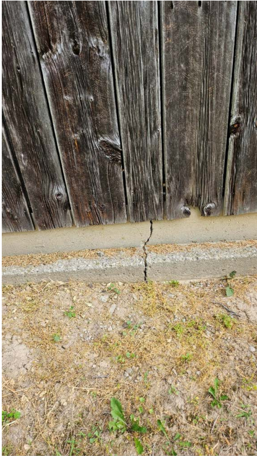
BUILDING 6 - FORBES BARN – FOUNDATION CRACK
