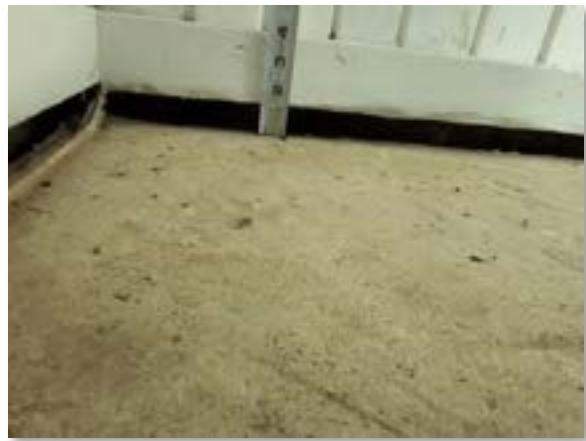
Image 77: Settled entry slab on grade
