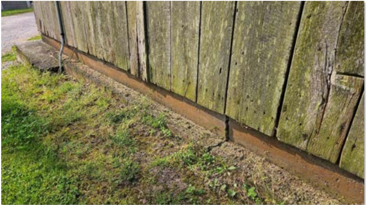
BUILDING 6 - FORBES BARN – FOUNDATION CRACK
