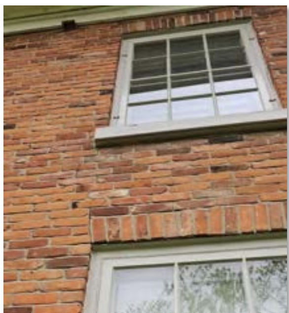
Image 8: Cracked brick at windows, typical.
