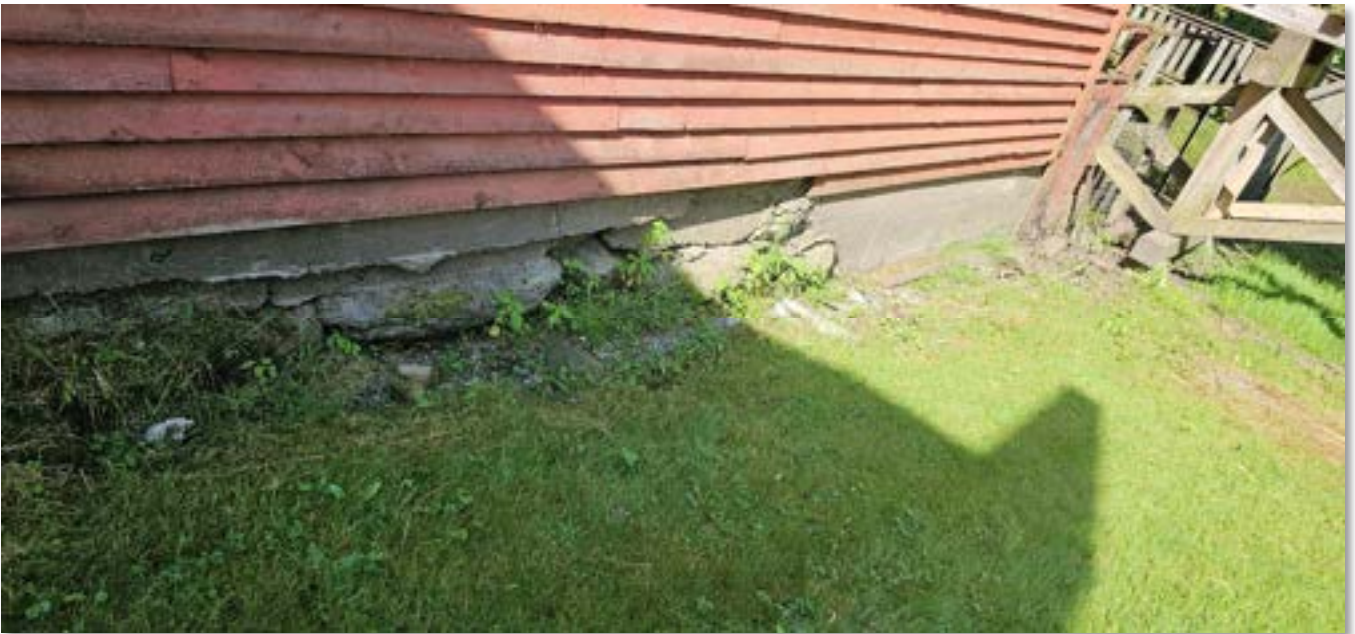
Image 1: Damaged foundation, North foundation wall.
