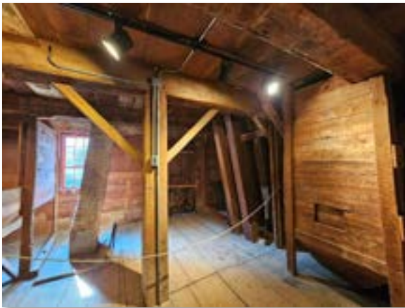
Image 19: Leaning Column – Main Floor
