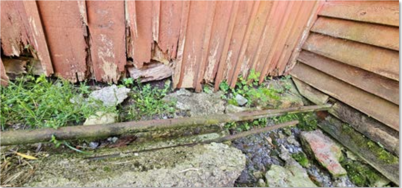
Image 4: Damaged wood, foundation and cladding, North extension.
