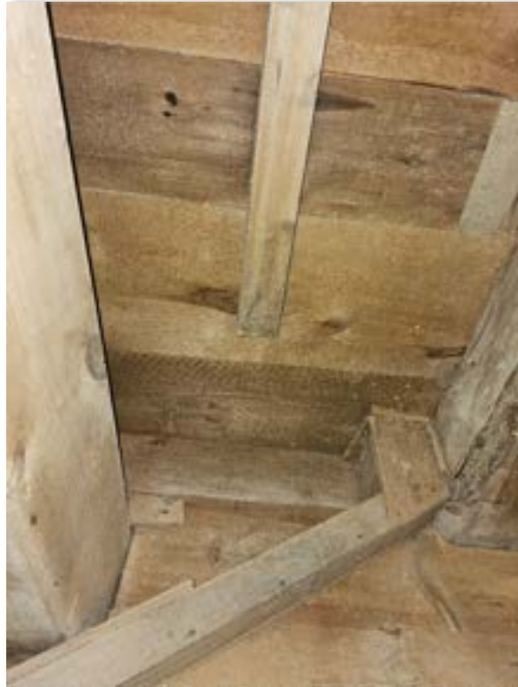
Image 14: Bending floor boards below equipment
