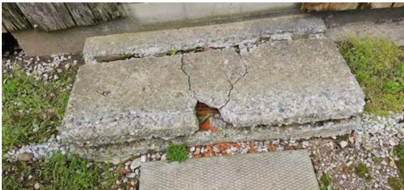
Image 18: Cracked concrete steps at entry
