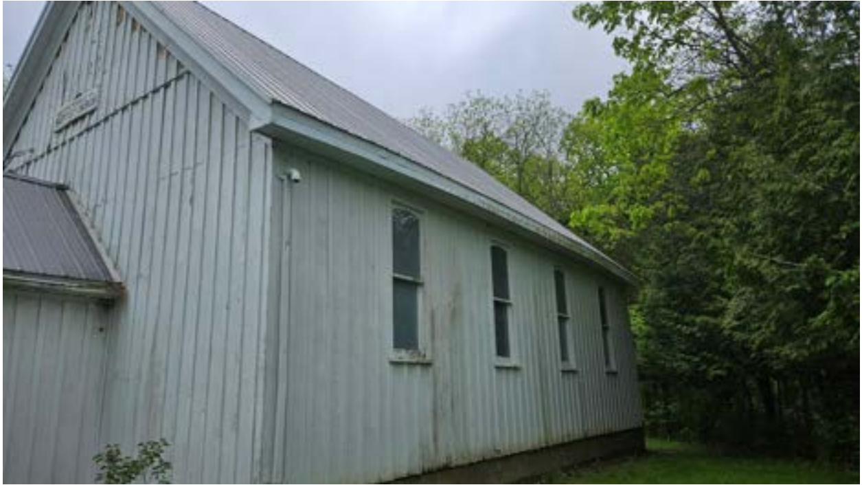
BUILDING 24 - TEETERVILLE CHURCH – BOWED EXTERIOR WALL
