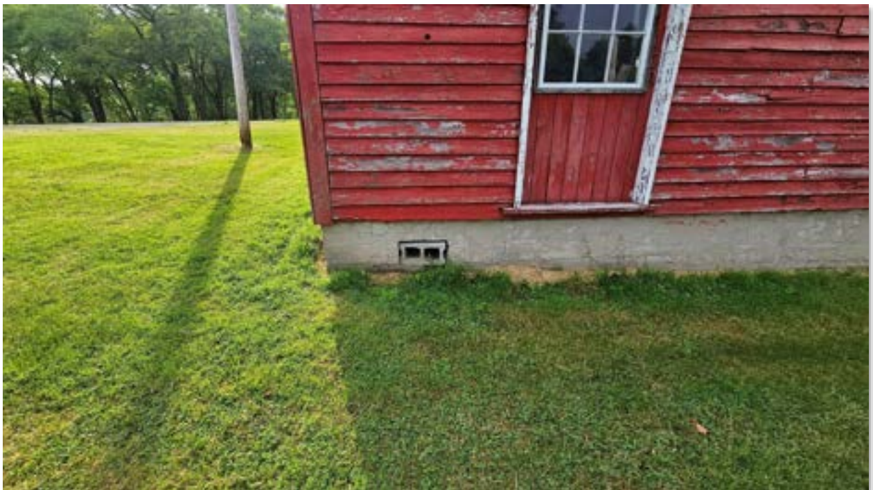
BUILDING 11 - VITTORIA CARRIAGE SHOP – HOLE IN FOUNDATION
