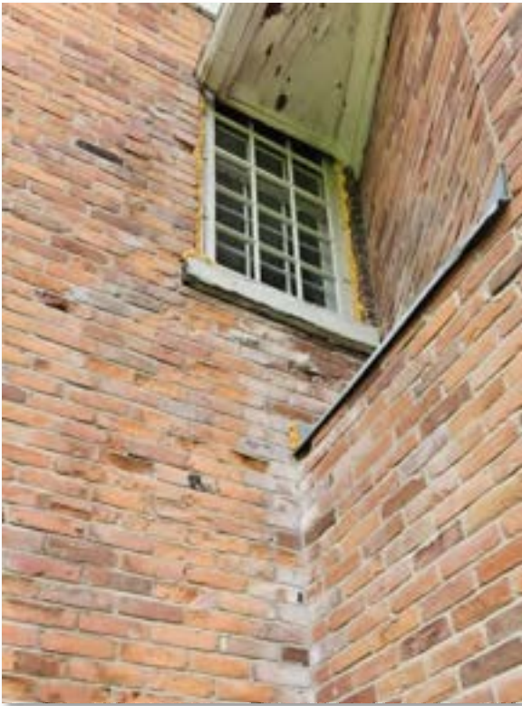
Image 6: Damaged Brick, Soffit and poor drainage at North side of building.
