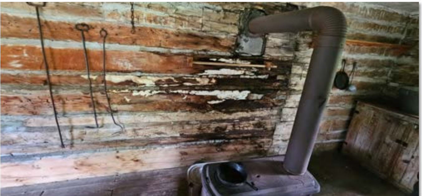
Image 60: Water penetrating into building around fireplace.
