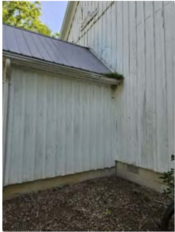
Image 71: blocked gutters.
