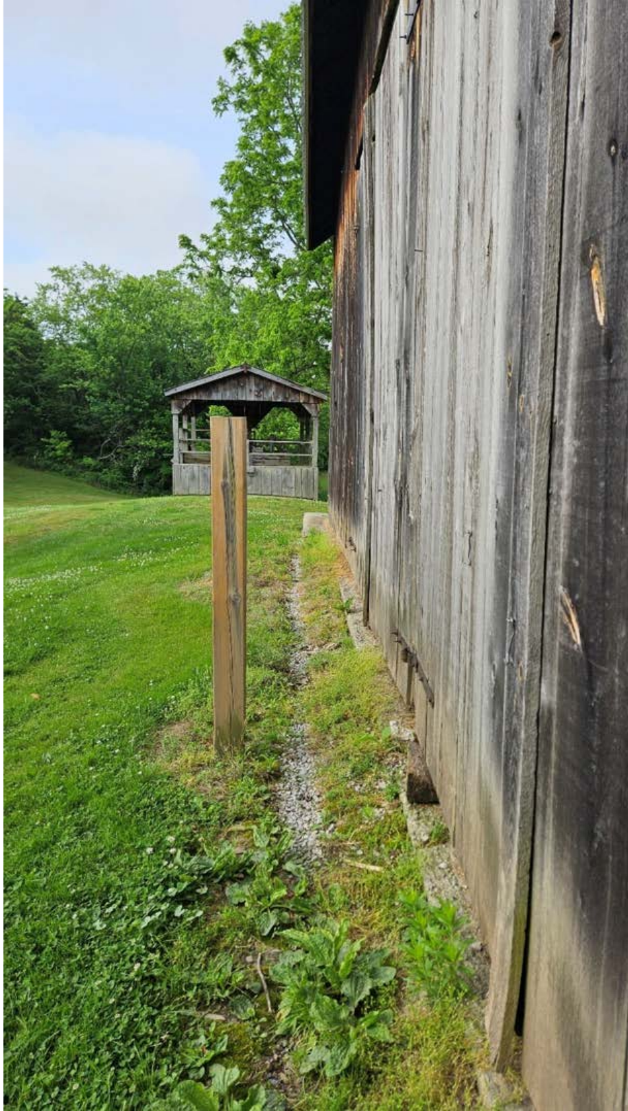
BUILDING 6 - FORBES BARN – ROOF DRIP TRENCH
