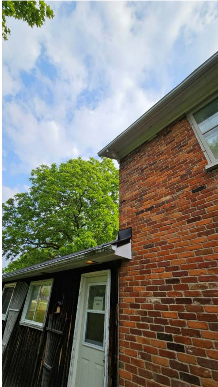
BUILDING 4 – HOMESTEAD – MISSING DOWNSPOUTS
