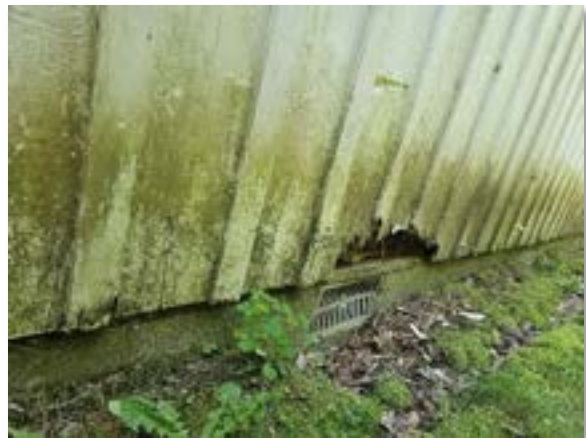
Image 73: Damaged Cladding moisture penetration
