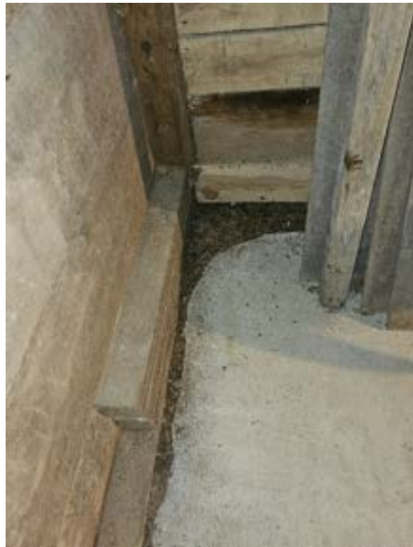
Image 30: Moisture at sunken North-East corner.
