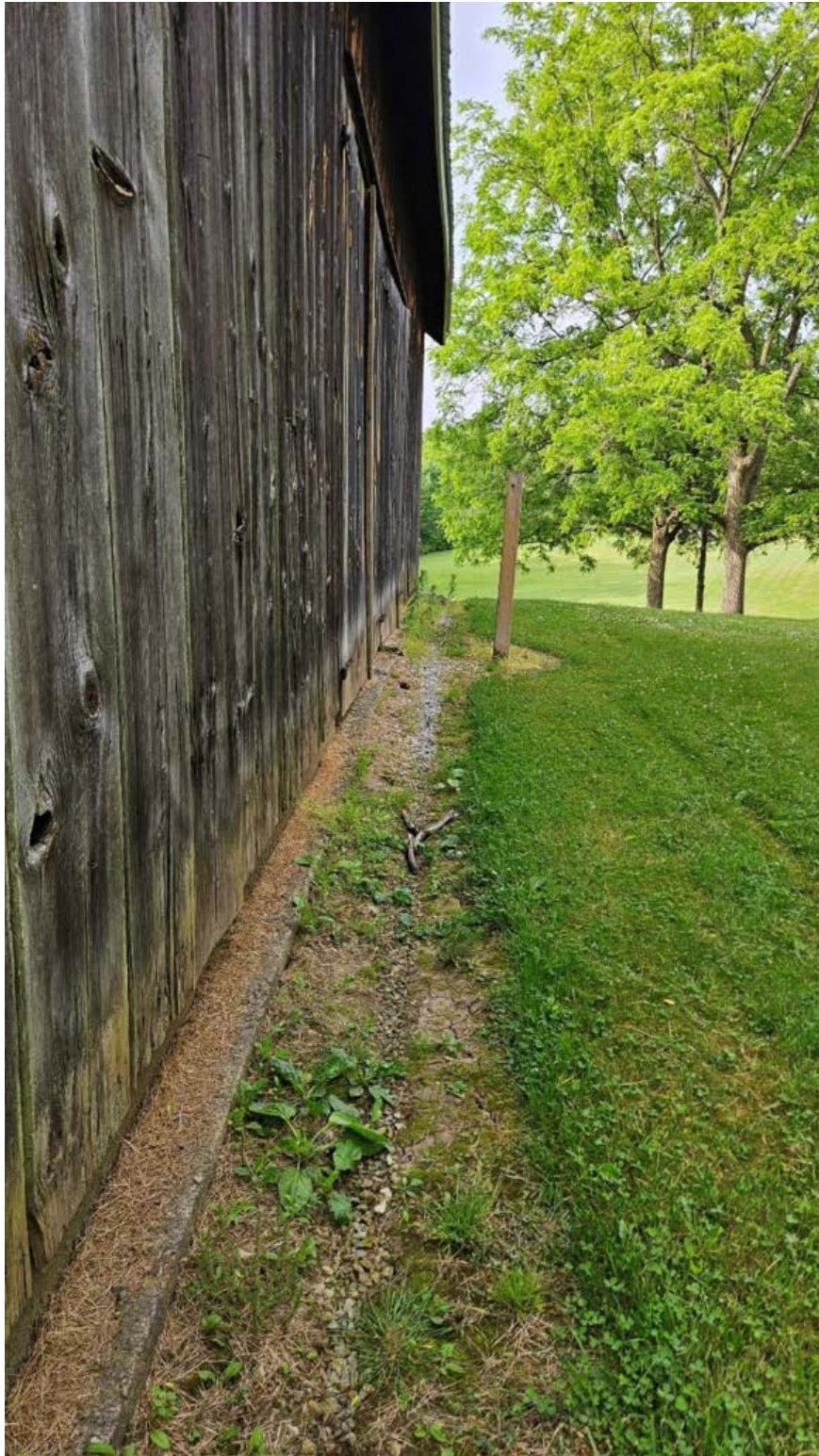
BUILDING 6 - FORBES BARN – ROOF DRIP TRENCH
