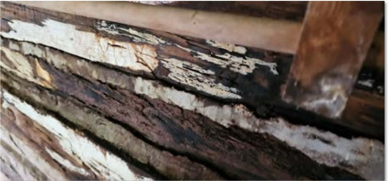
Image 62: Water penetrating into building around fireplace.
