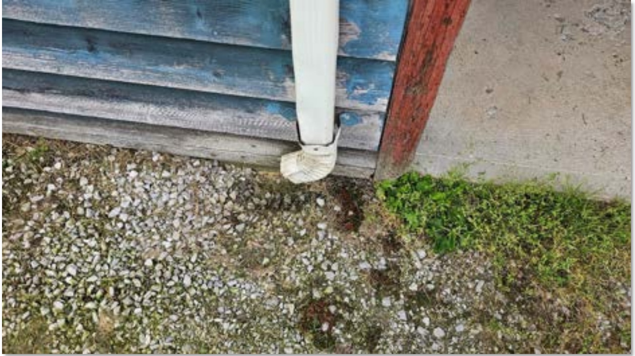
BUILDING 14 – STOREFRONTS - IMPROPER DRAINAGE
