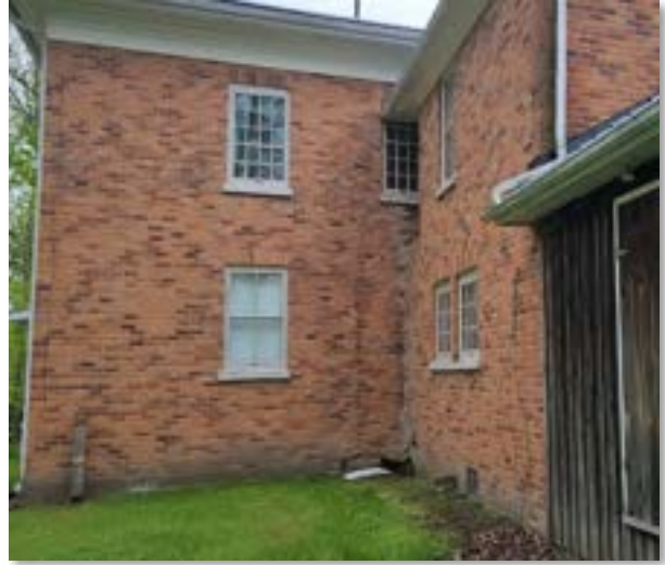
Image 5: Damaged Brick, Soffit and poor drainage at North Side of building.
