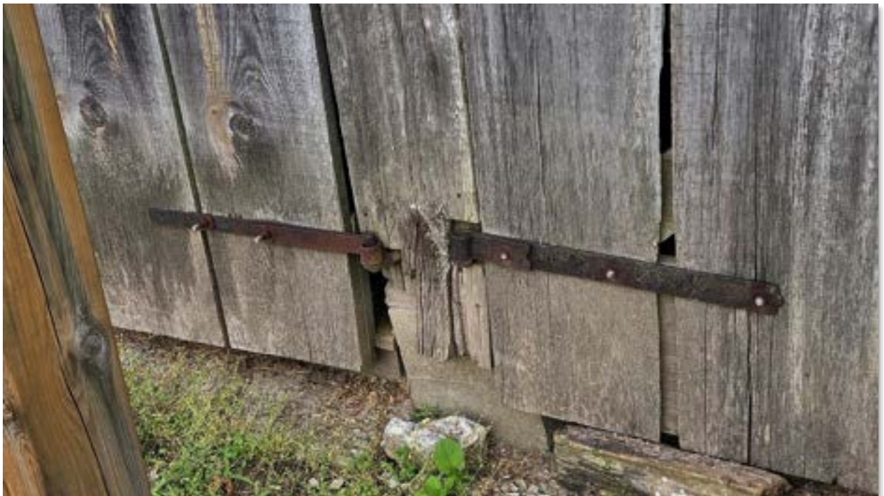
BUILDING 6 - FORBES BARN – FAILING HARDWARE
