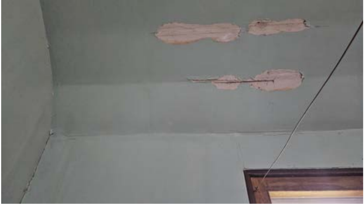
BUILDING 24 - TEETERVILLE CHURCH - INTERIOR WATER DAMAGE
