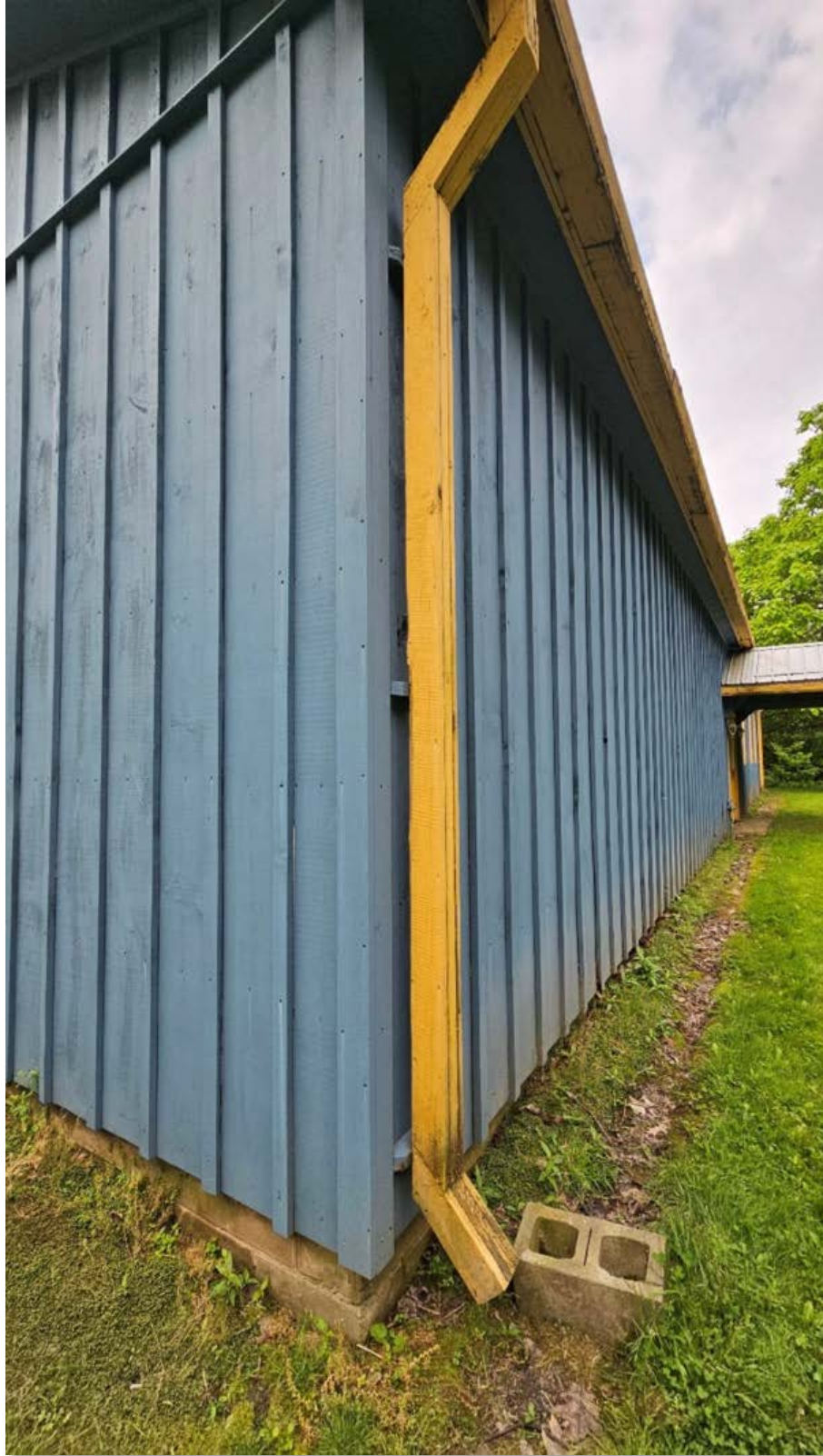
BUILDING 8 – MUSEUM – WOODEN DOWNSPOUT AND EROSION
