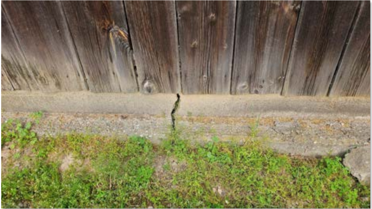
BUILDING 6 - FORBES BARN – FOUNDATION CRACK
