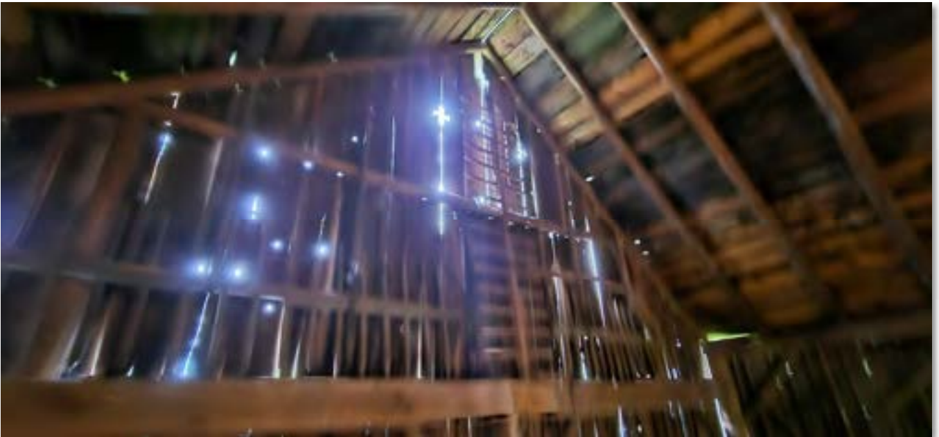
Image 20: Typical gable end wall and roof framing.
