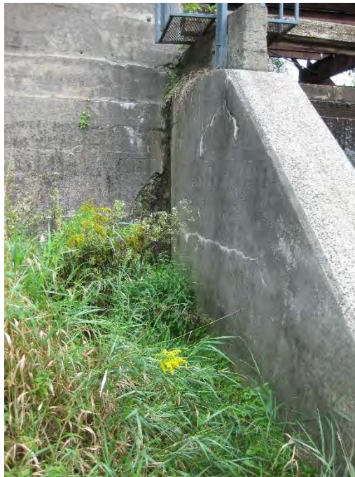
Photo 8: Looking north at northwest downstream wingwall Note: Seepage between concrete wingwall and pier
