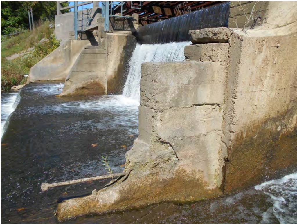
Photo 4: Concrete Deterioration at Middle Pier
