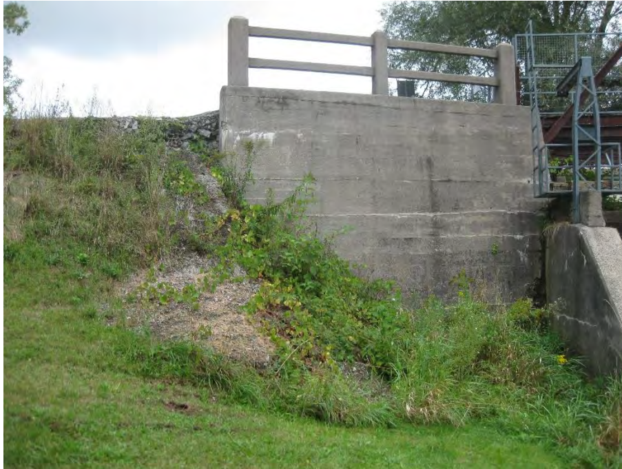
Photo 7: Looking north at northwest downstream wingwall Note: material loss at top corner; Slump at bottom of slope
