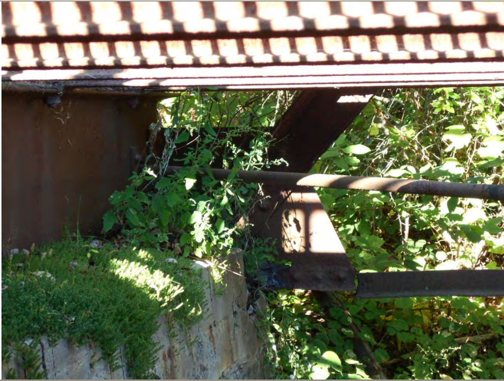
Photo 13: Failed Bottom Chord
