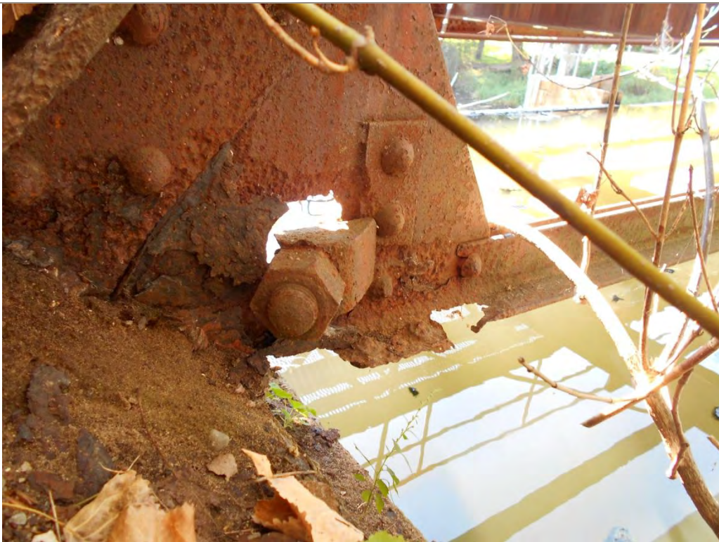
Photo 12: Deterioration at Connection
