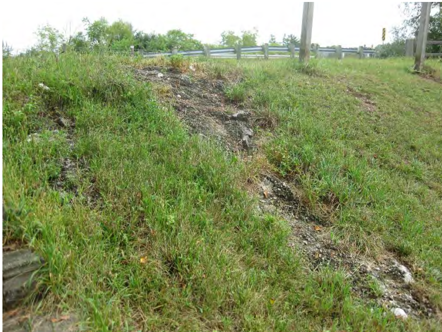
Photo 6: Looking north at northwest downstream slope Note: Close up image of erosion
