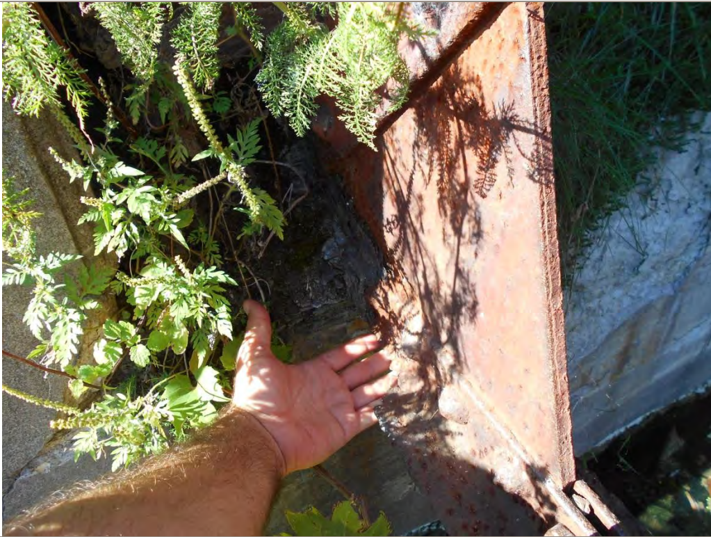
Photo 11: Loss of Section at Connection
