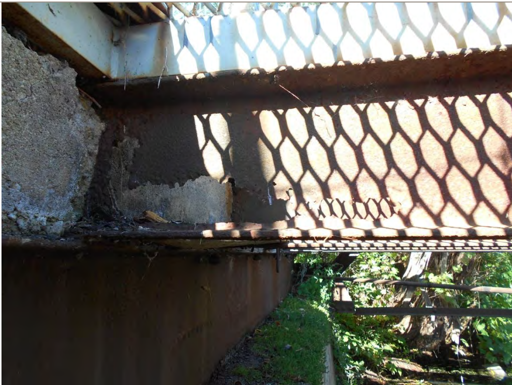
Photo 10: Loss of Web Section in Stringer
