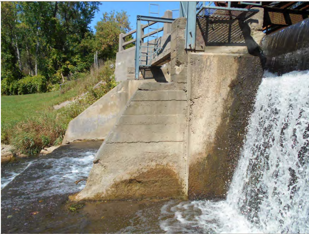
Photo 5: Scaling at North Pier
