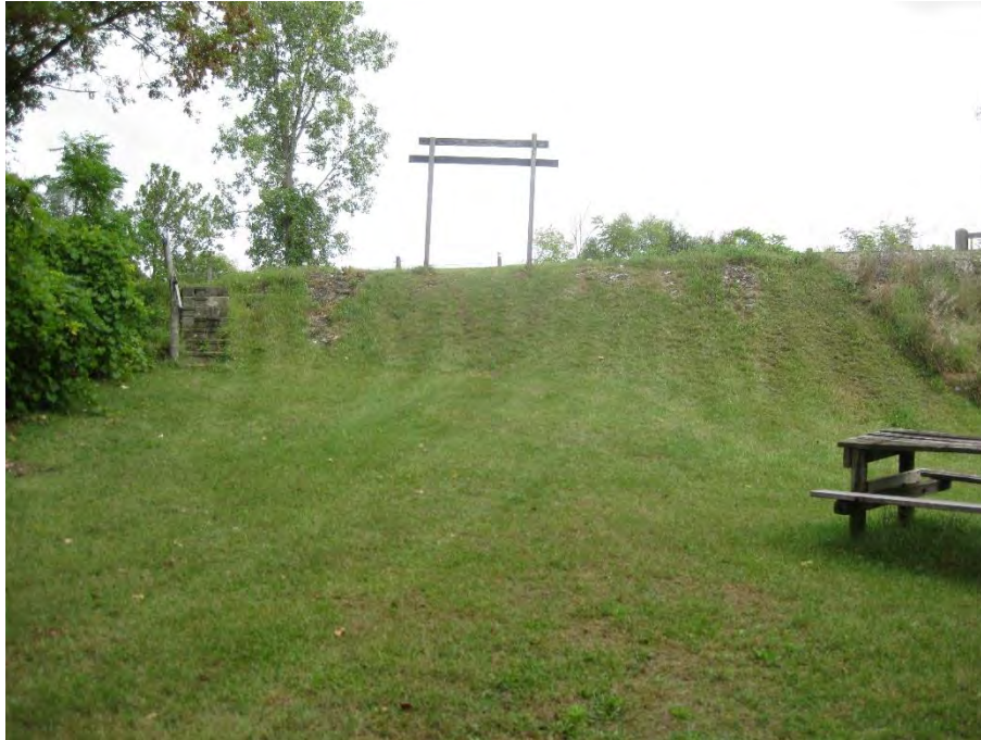
Photo 5: Looking north at northwest downstream slope Note: Eroded patches in the grass due to run-off
