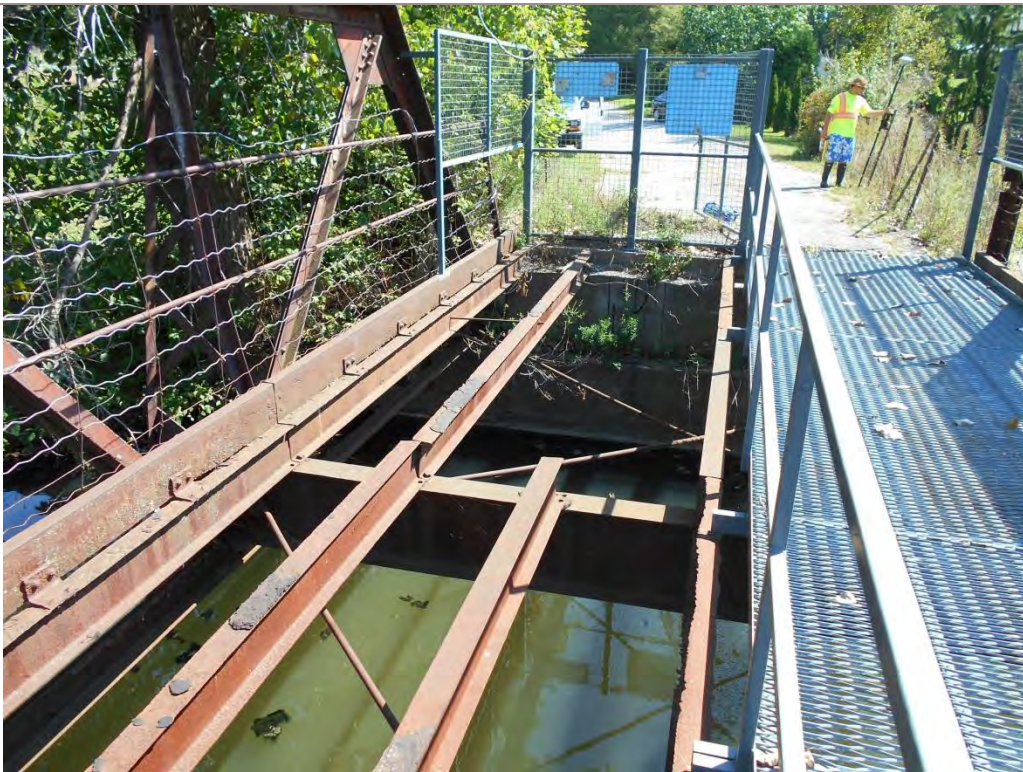
Photo 8: Missing Stringer on Bridge
